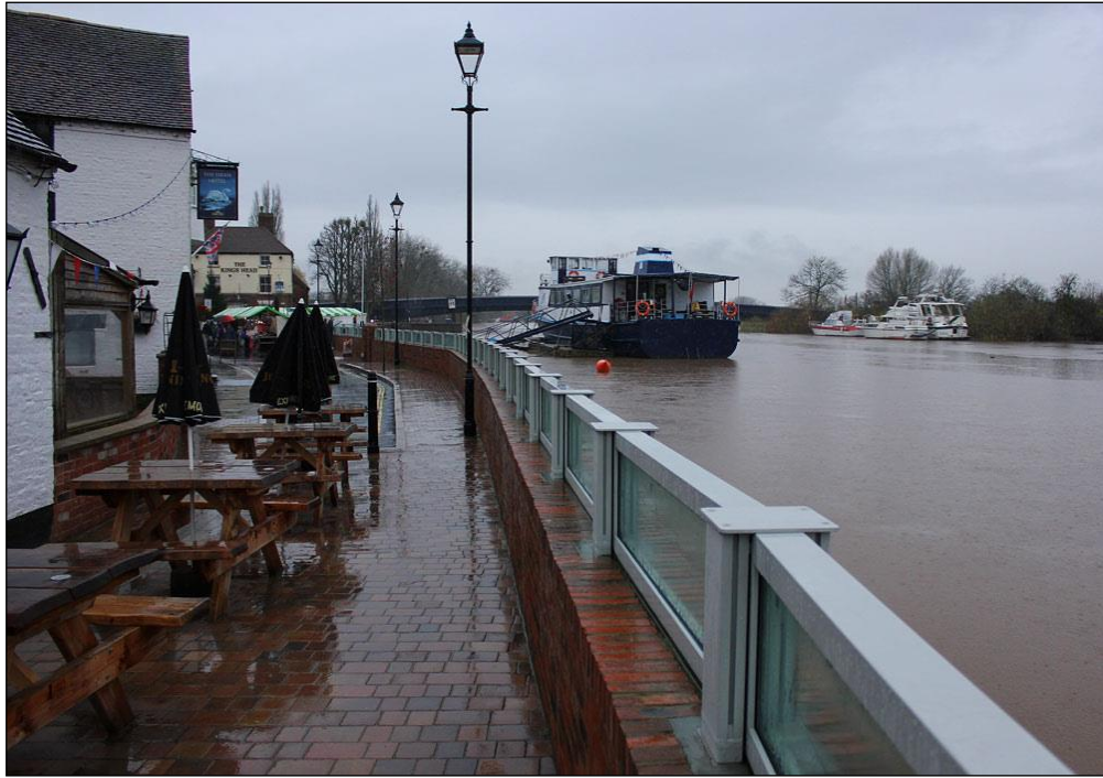
Figure 6.2: Upton-Upon-Severn flood defence (Copy rights Environment Agency).
