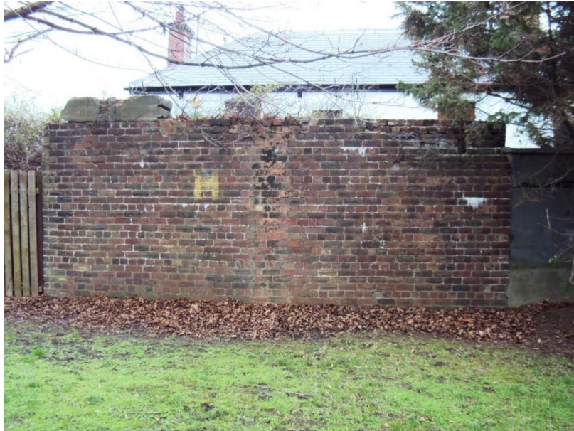
Figure 119: Winding engine support, California (Source: Author)
