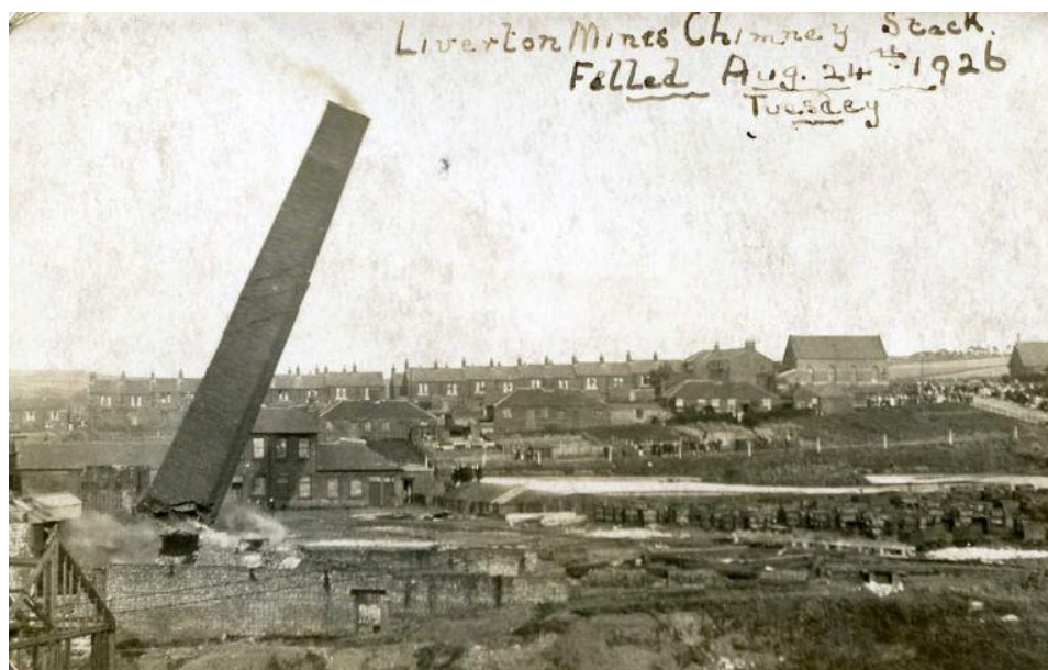
Figure 90: Demolition on the mine site (Source: Author)
