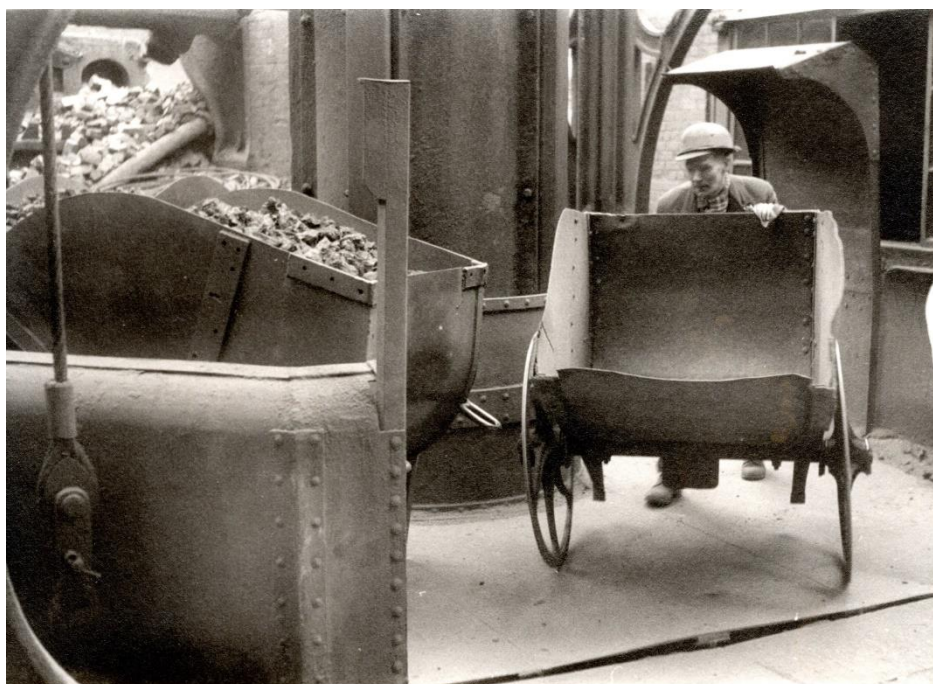
Figure 2: Charging barrows on the blast furnace pneumatic hoist table (Source: CIAS Archive)
