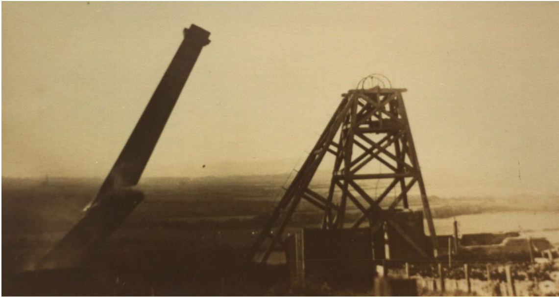
Figure 34: The demolition of the Brotton Mine chimney (Source: Author)
