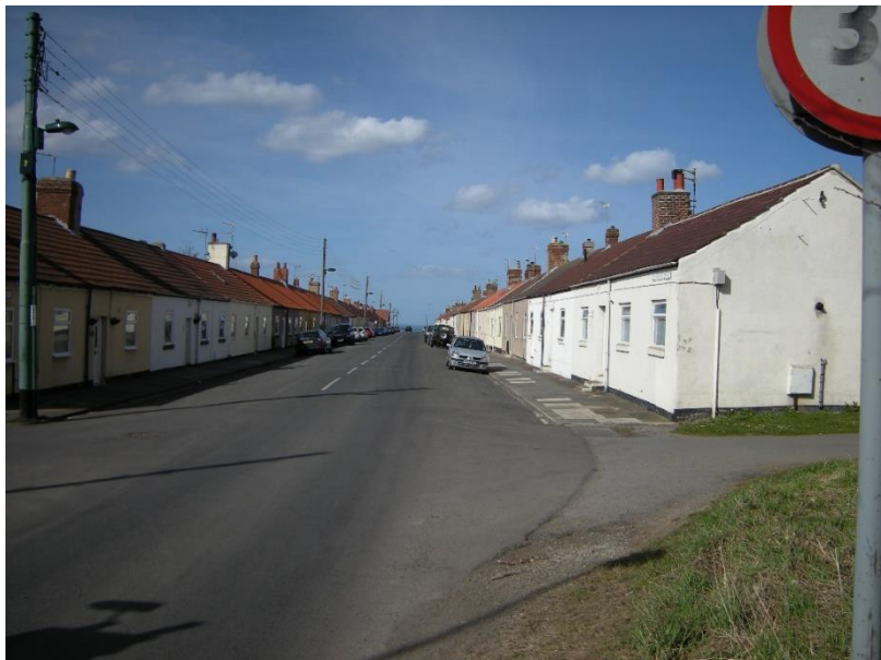
Figure 108: Cleveland Street (Source: Author)
