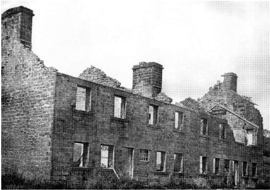
Figure 69: West Mine housing (Source: Simon Chapman, Cleveland Ironstone Mines: Old Pictures Volume 4: Rosedale Mines and Railway (Guisborough: Peter Tuffs, 2007), 50)
