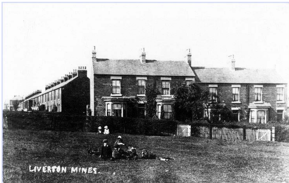
Figure 62: Cliffe Terrace and Liverton Terrace (Source: East Cleveland Image Archive)
