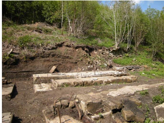
Figure 18: The Grinkle Mine engine house foundations (Source: Author)
