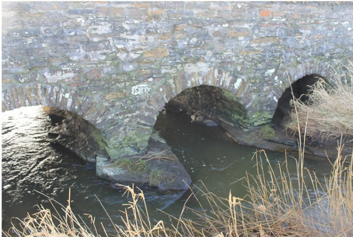
Figure 6 a) Bridge at centre of Douby transect showing piers founded on bedrock, b) stream channel cut into bedrock
