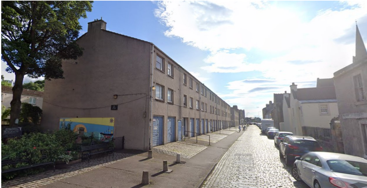
Figure 7.17. Newhaven Comprehensive Redevelopment Area by Ian G Lindsay & Partners, showing fisherman's stores built into the ground floor of the new flats.
