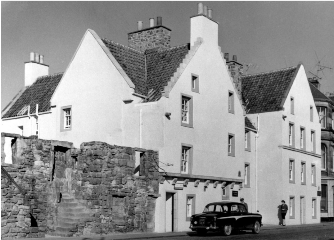
Figure 3.6. Wheeler & Sproson's Offices at Sailor's Walk, Kirkcaldy, taken shortly after its 1954 to 1959 restoration.
