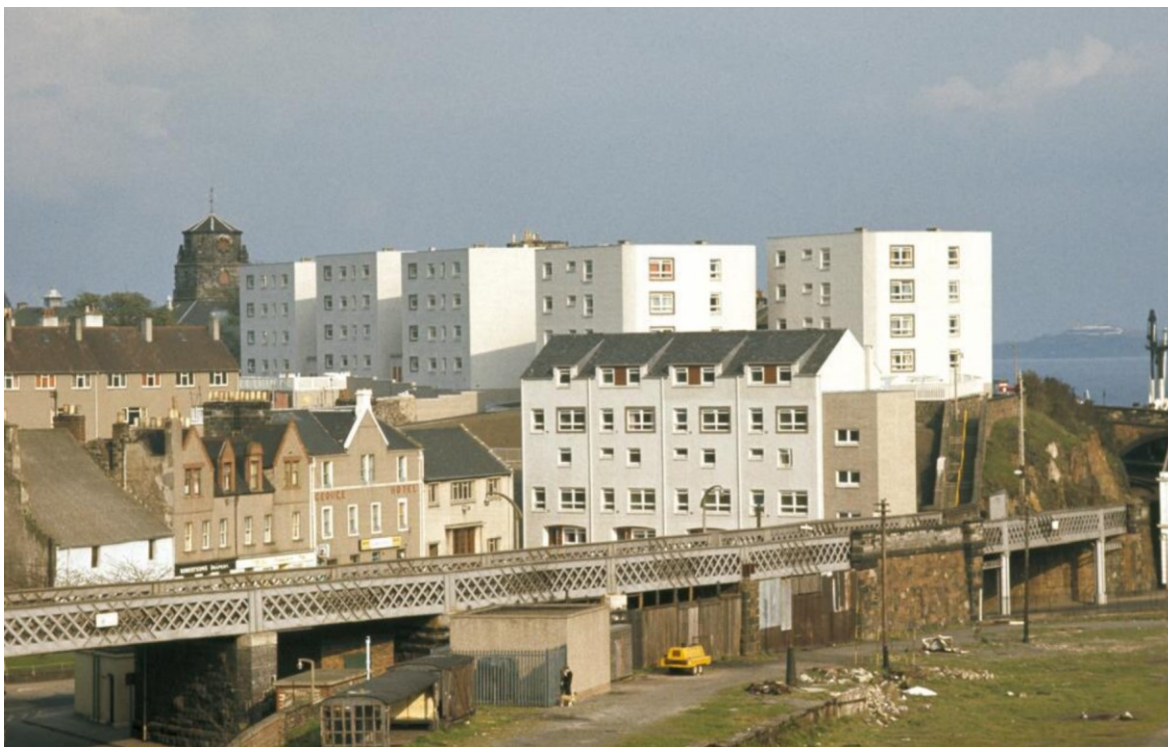
Figure 6.8. View of West Leven Street from Rossend Castle showing all six blocks of the West Leven Street development, highlighting the relationship between the two hill sites.
