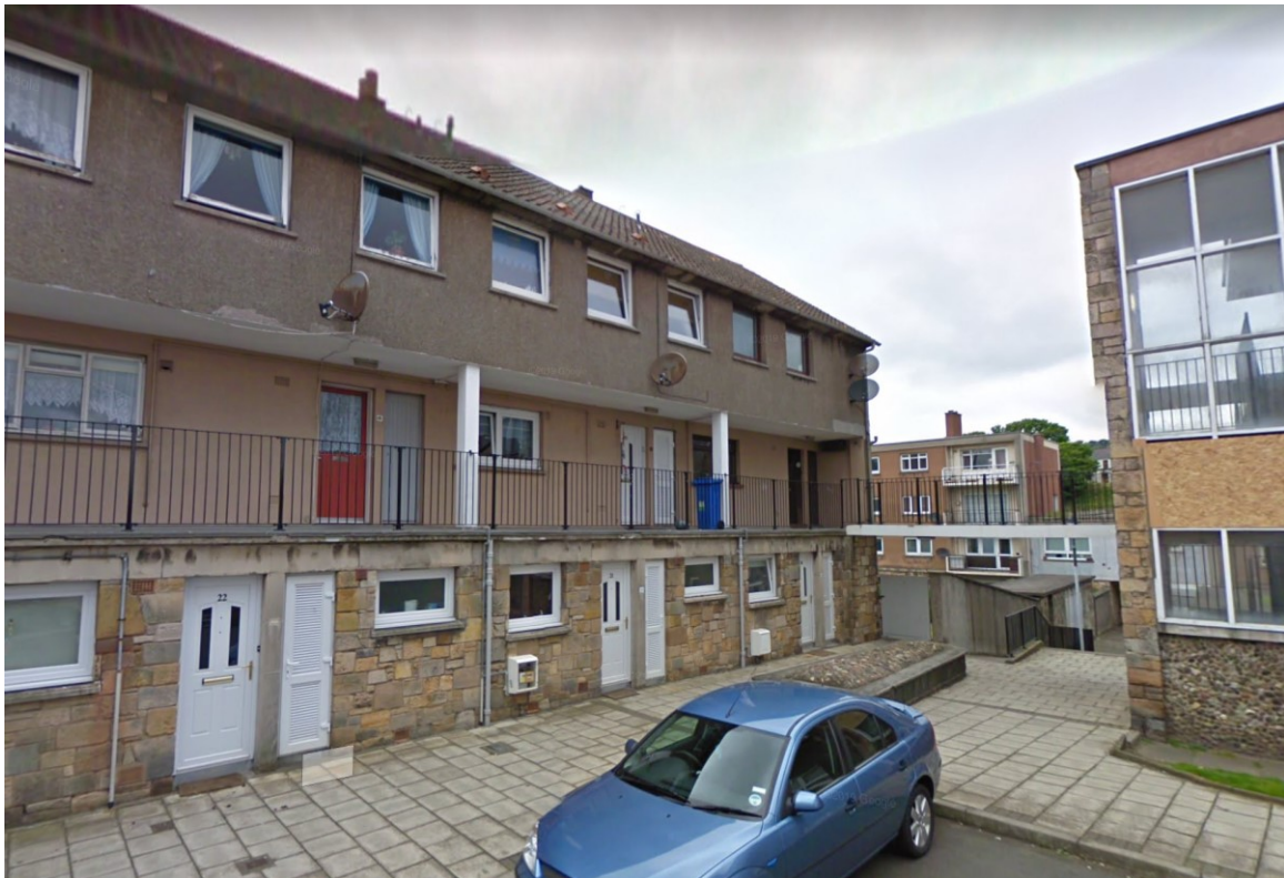
Figure 6.15. A combination of rubble masonry, harling and pantiles is used at Burntisland's Somerville Street/ High Street Development.
