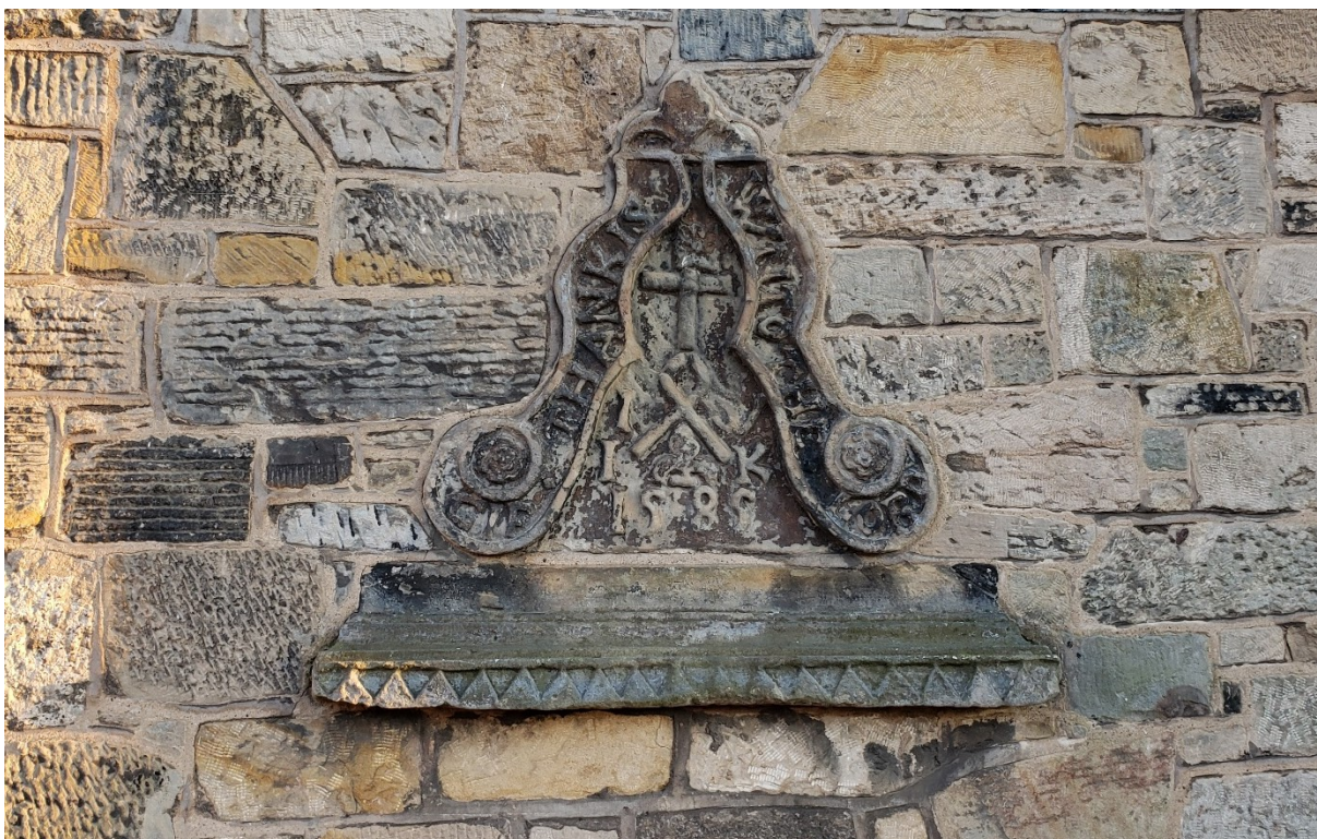
Figure 6.14. Example of a marriage lintel dating from 1585 used within the new buildings at Dysart's Phase 1, Block D.
