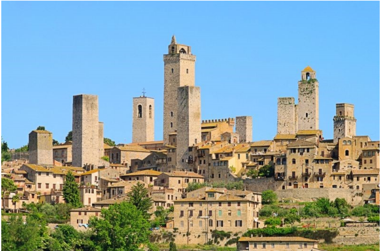
Figure 6.30. The Towers of San Gimignano in Tuscany date from the 13 th century and are quoted as being an influence for Wheeler & Sproson's small residential towers.
