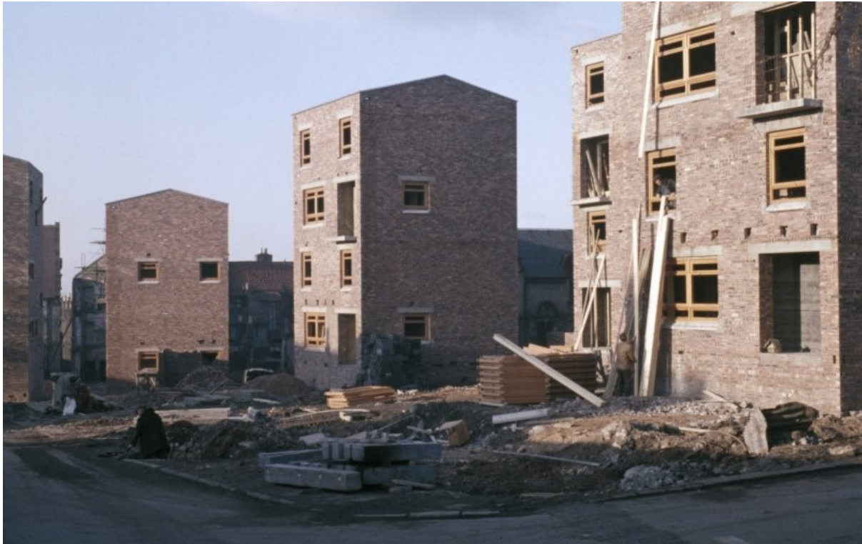
Figure C.10. The brick structure of Wheeler & Sproson’s small tower blocks in Dysart Phase 2 is clearly shown in this photograph from their construction. In some respects, they arguably share a similarity to the modern Colonies discussed above.
