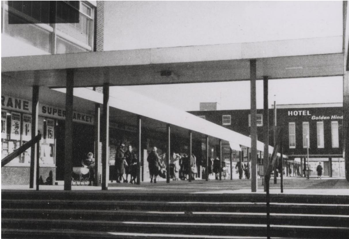
Figure 7.38. Blackburn Shopping Centre by Wheeler & Sproson, since demolished.
