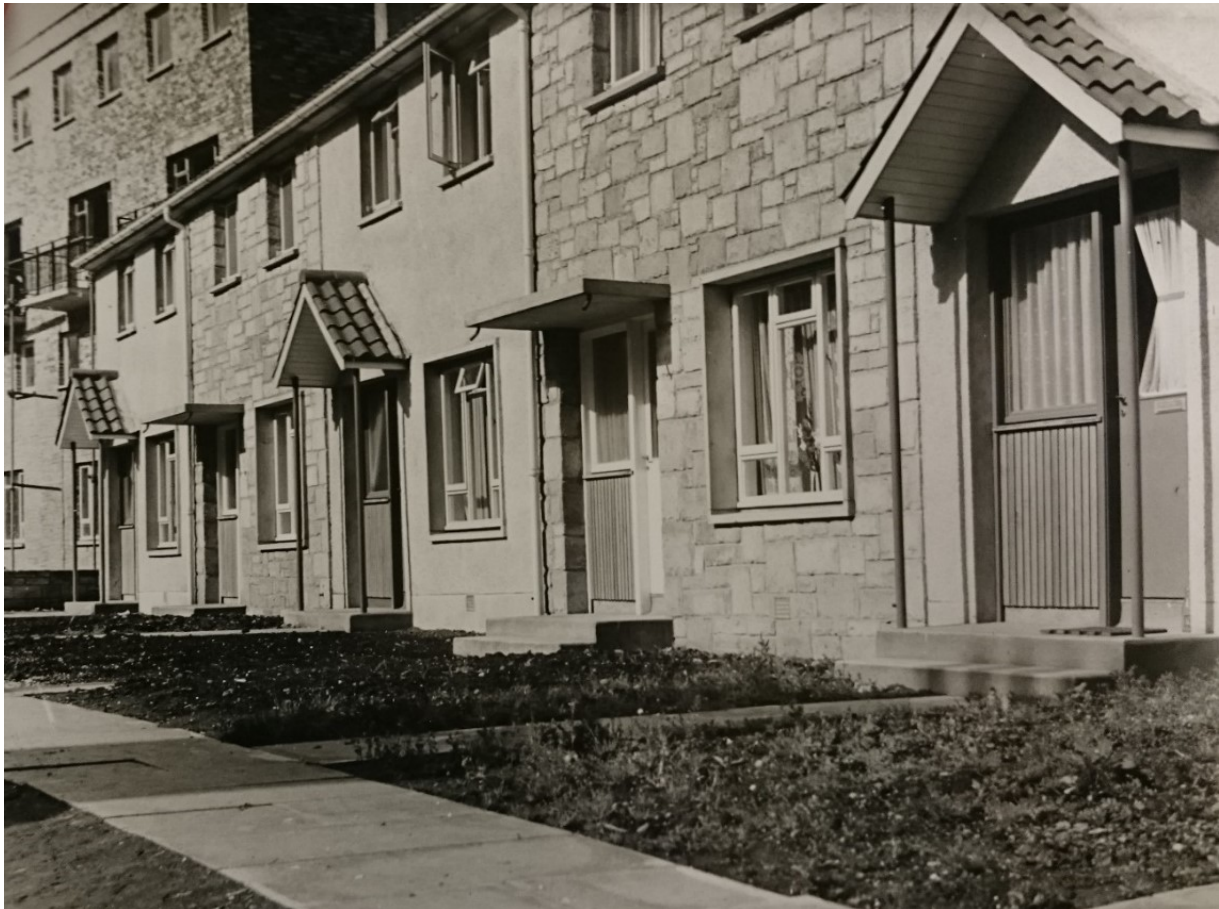
Figure 4.11. The terraced houses on Somerville Square (Block B4) used contrasting finishes to create a sense of individuality, undated.
