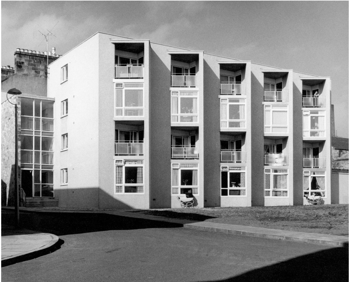
Figure 6.32. The 'Zig-Zag' flats in Dysart were the first of their kind used by Wheeler & Sproson. They faced on to a landscaped green where families appear to have left their prams with babies inside!
