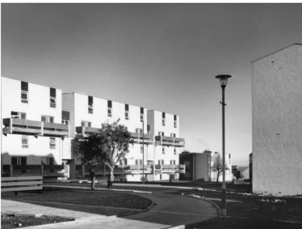
Five-storey deck access slab block at Dysart Phase 2
