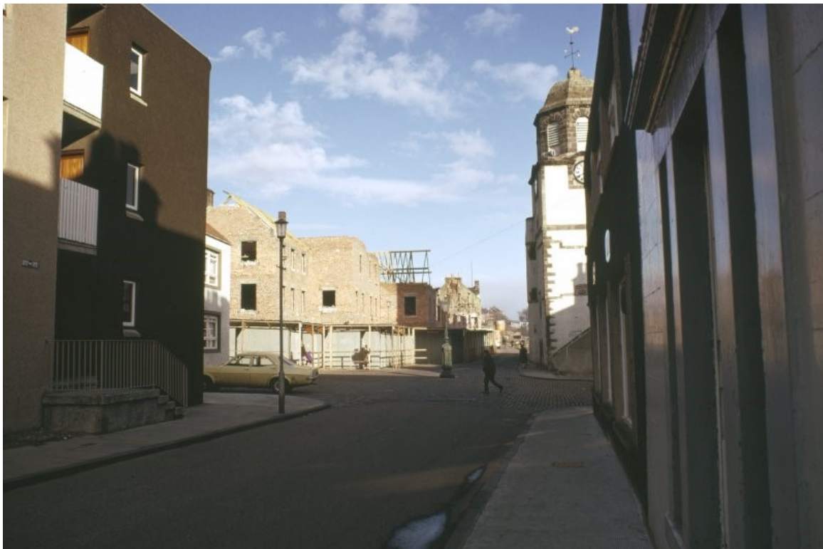
Figure 5.53. 43-67 High Street, Dysart during construction, showing the brick and timber structure employed, circa 1971.
