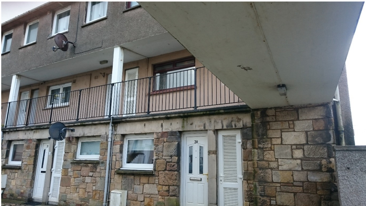
Figure 6.27. Three of the four bands of colour and texture used at Somerville Street/ High Street can be seen here, creating a horizontally emphasised block.
