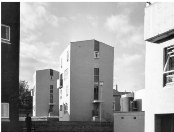
Four of the six small towers of Dysart Phase 2
