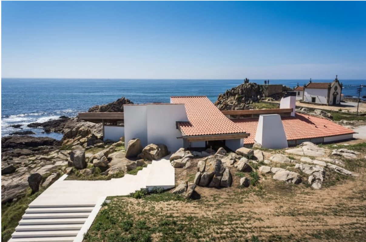
Figure 2.9. The Boa Nova Tea House, Matosinhos, Portugal. It was designed in 1956 by Fernando Távora and Álvaro Siza Vieira, making use of local white plastered masonry walls and pantiles, alongside red African ‘Afizelia’ wood in the cladding of the walls.
