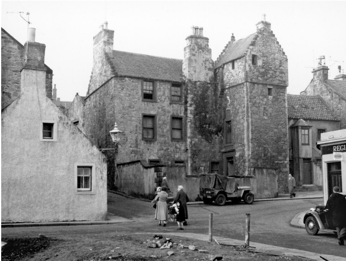
Figure 5.47. 'The Towers' in Dysart taken prior to restoration, circa 1962.
