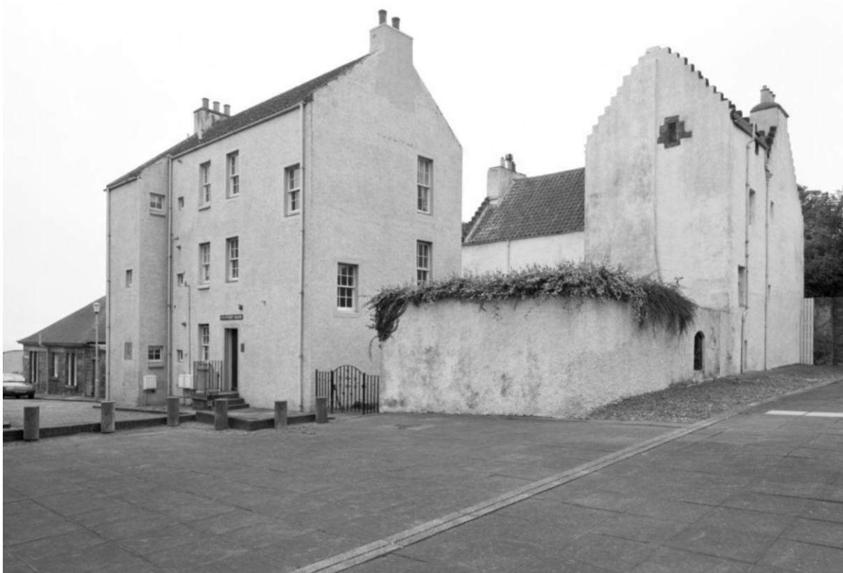
Figure 6.11. The high-walled courtyard of St. David’s, Dysart, with Phase 2 – Part 1, Block 2 forming one side of the square (to the left). Gateways and portals in the courtyard wall provide views out to the surrounding area.
