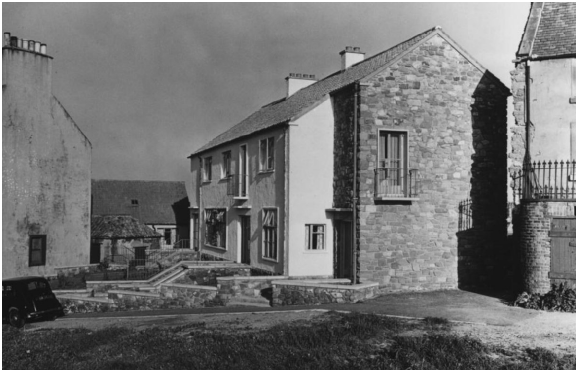
Figure 2.4. The low front garden walls at Spence's Dunbar development, seen here, were viewed by McWilliam as unsuitable for the character of the area. Image taken in 1952.
