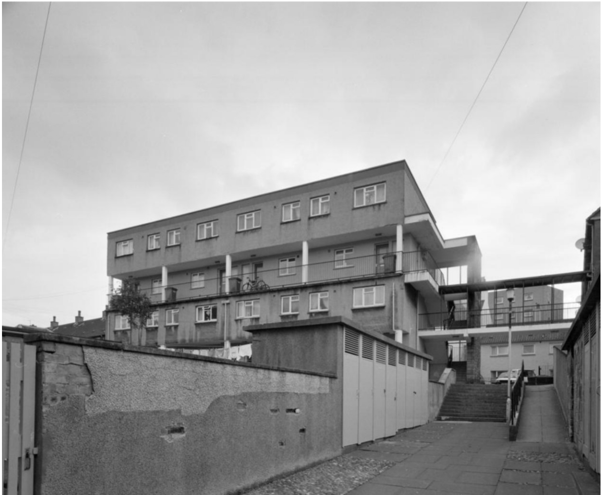
Figure 6.34. Photograph of the rear of Somerville Street/ High Street block 'B3' showing the access bridge linking to Block 'B2' and the semi-exposed stairwell tower.
