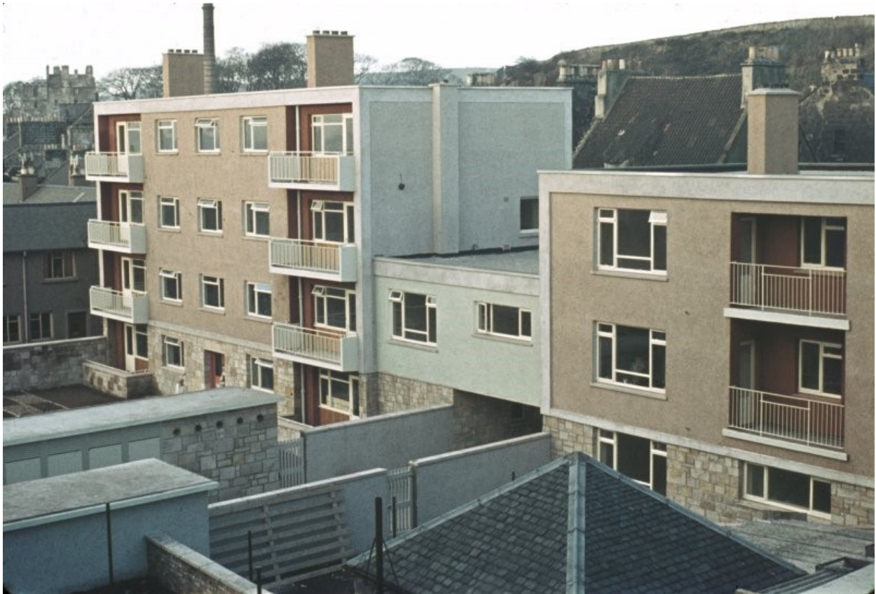
Figure 4.12. High Street blocks (B1) linked by a first storey connecting section containing a two bedroom flat, over a pend and pram stores, undated.
