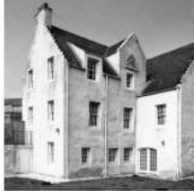
4) Restoration of 'The Anchorage' Dates: 1963—1967
