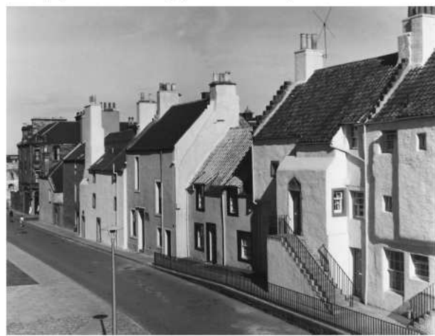
Image of Burntisland's Somerville Street after restoration.
