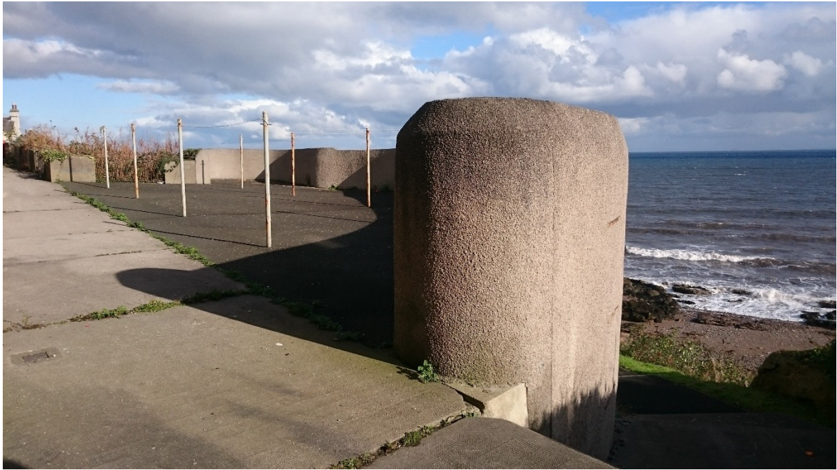
Figure 6.2. The existing stone retaining wall was incorporated into Dysart Phase 1, Block D and used as a drying green.
