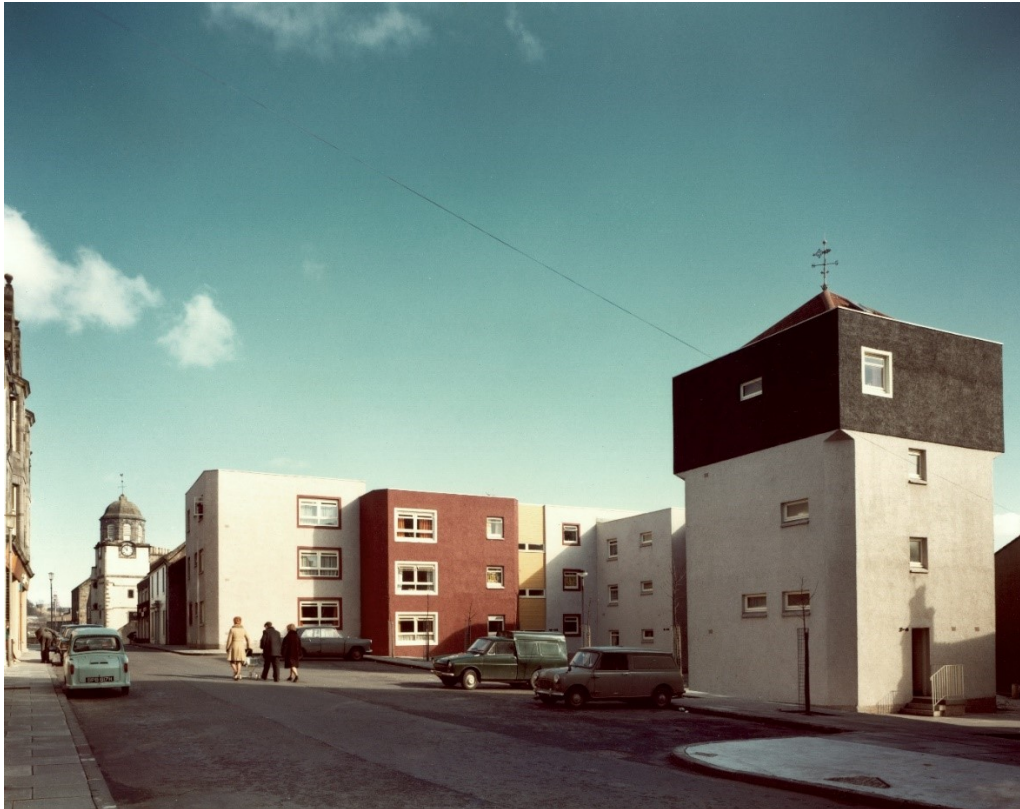
Figure 5.30. Dysart Phase 3 – Part 1, Blocks 5, 6, 7 and 8, circa 1973. The octagonal tower of the Tollbooth can be seen to the left side of the image.
