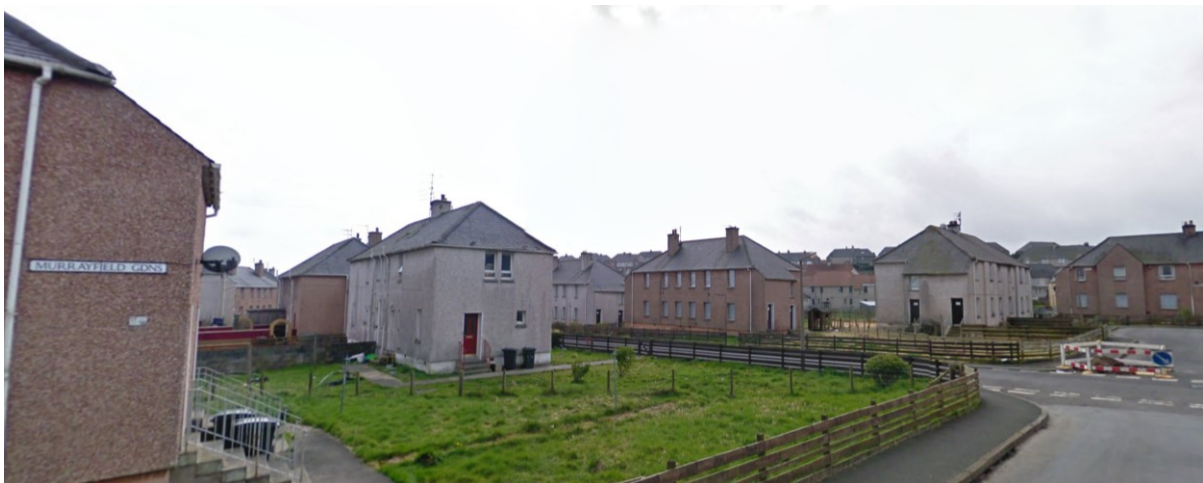
Figure 3.2. Dick's Hill development by Alexander Maclean Goudie, built 1937.
