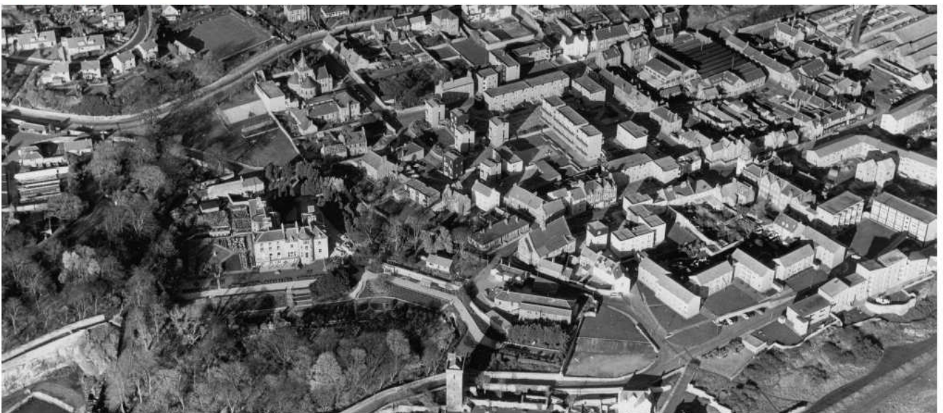
Aerial Photograph of Dysart Redevelopment Project Circa 1975
