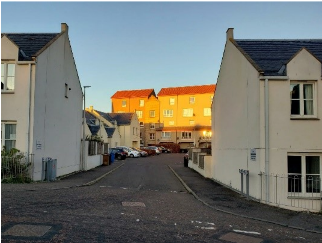
Figure C.14. The cul-de-sac which replaced large areas of the Fitzroy Square area of Wheeler & Sproson’s Dysart Redevelopment, with the much-altered Phase 2, Block 5 acting as a backdrop.
