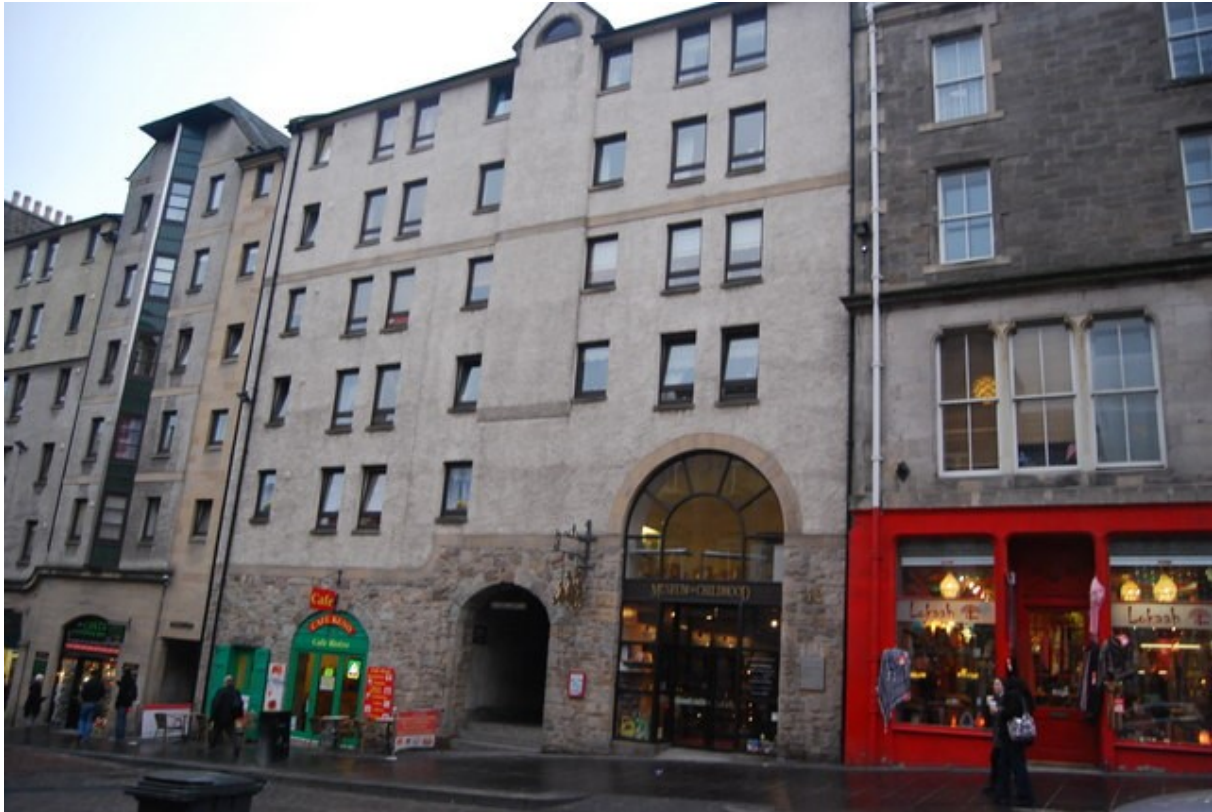
Figure 7.35. Museum of Childhood by Wheeler & Sproson, with their sheltered housing development to the left hand side of the image.
