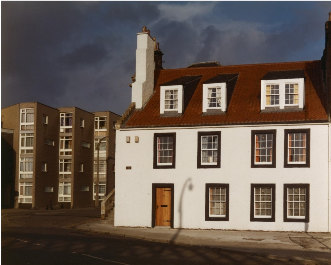
Figure 4.50. Image showing a completed 1-2 Harbour Place (Job 672) with the High Street/ Lothian Street (Job 178) block 'P' behind, circa 1975.
