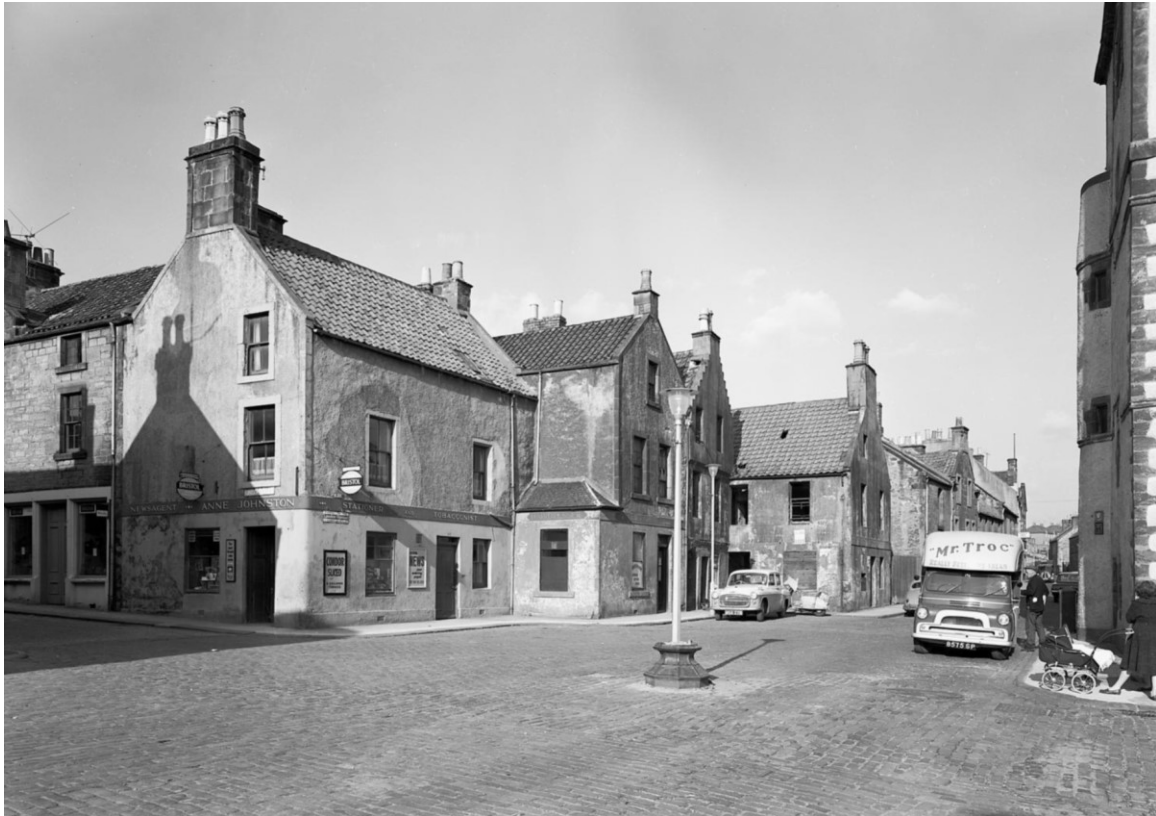
Figure 5.52. 43-67 High Street prior to reconstruction by Wheeler & Sproson, taken 1964.
