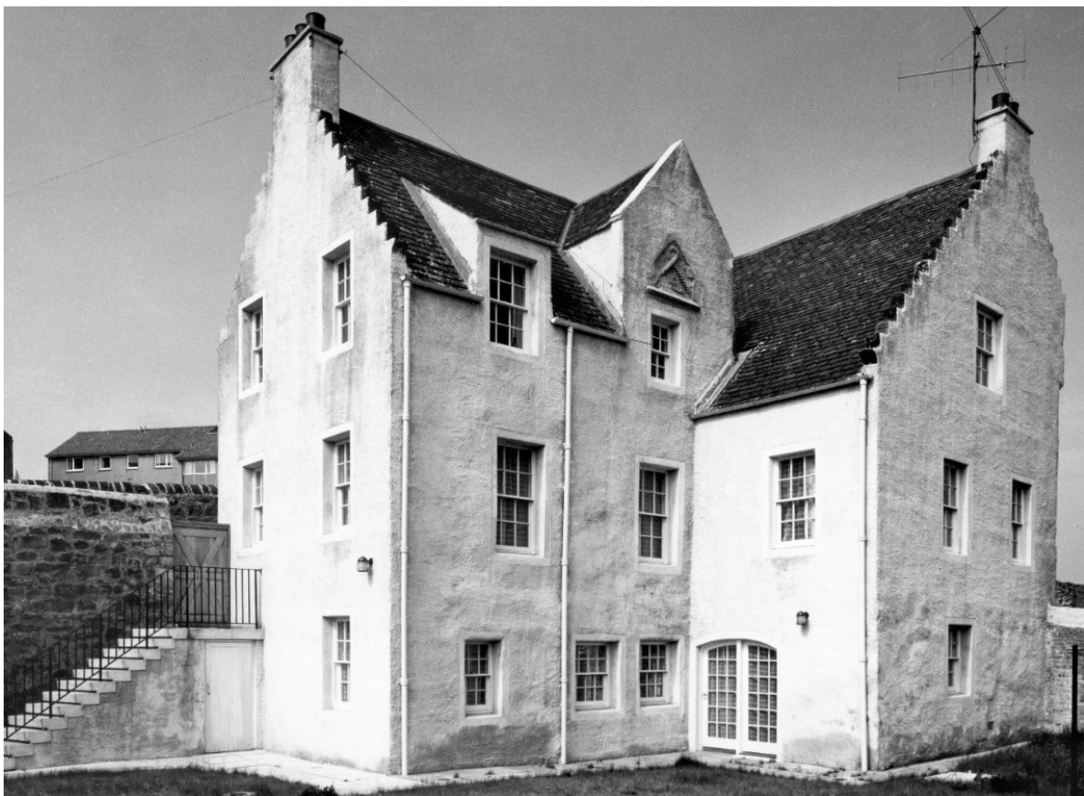
Figure 5.51. The Anchorage post restoration work, circa 1967. Block A of Phase 1 can be seen behind.
