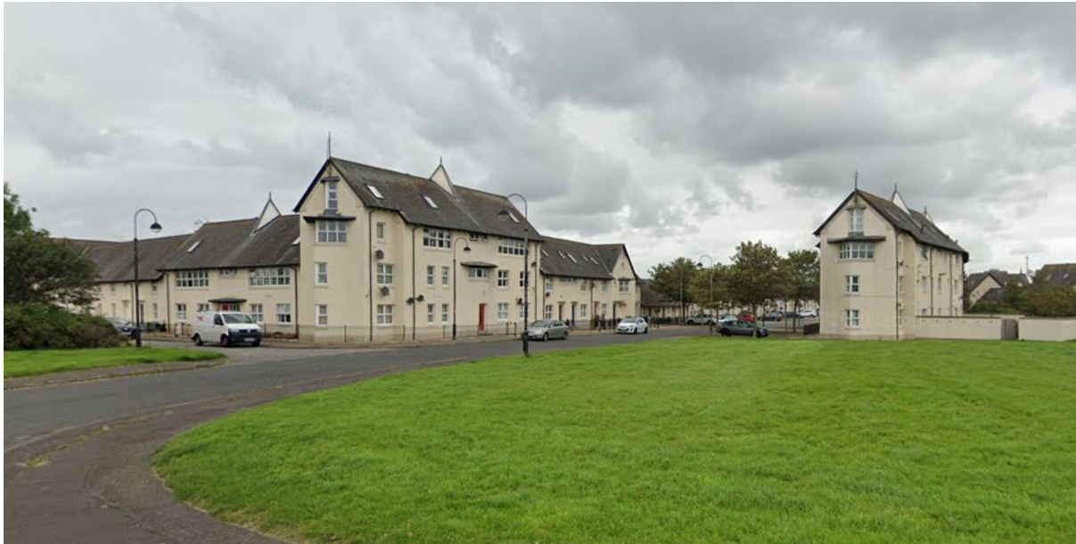
Figure C.4. Roan Rutherford's Peter Street and Gottries Crescent developments blended traditional harling and slates with an unusual, jagged use of glazing.
