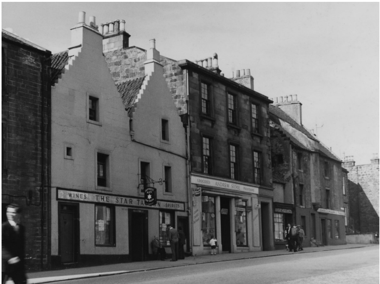
Figure 4.46. 41 High Street (Job 368) and the 'Star Tavern', shown here prior to restoration.
