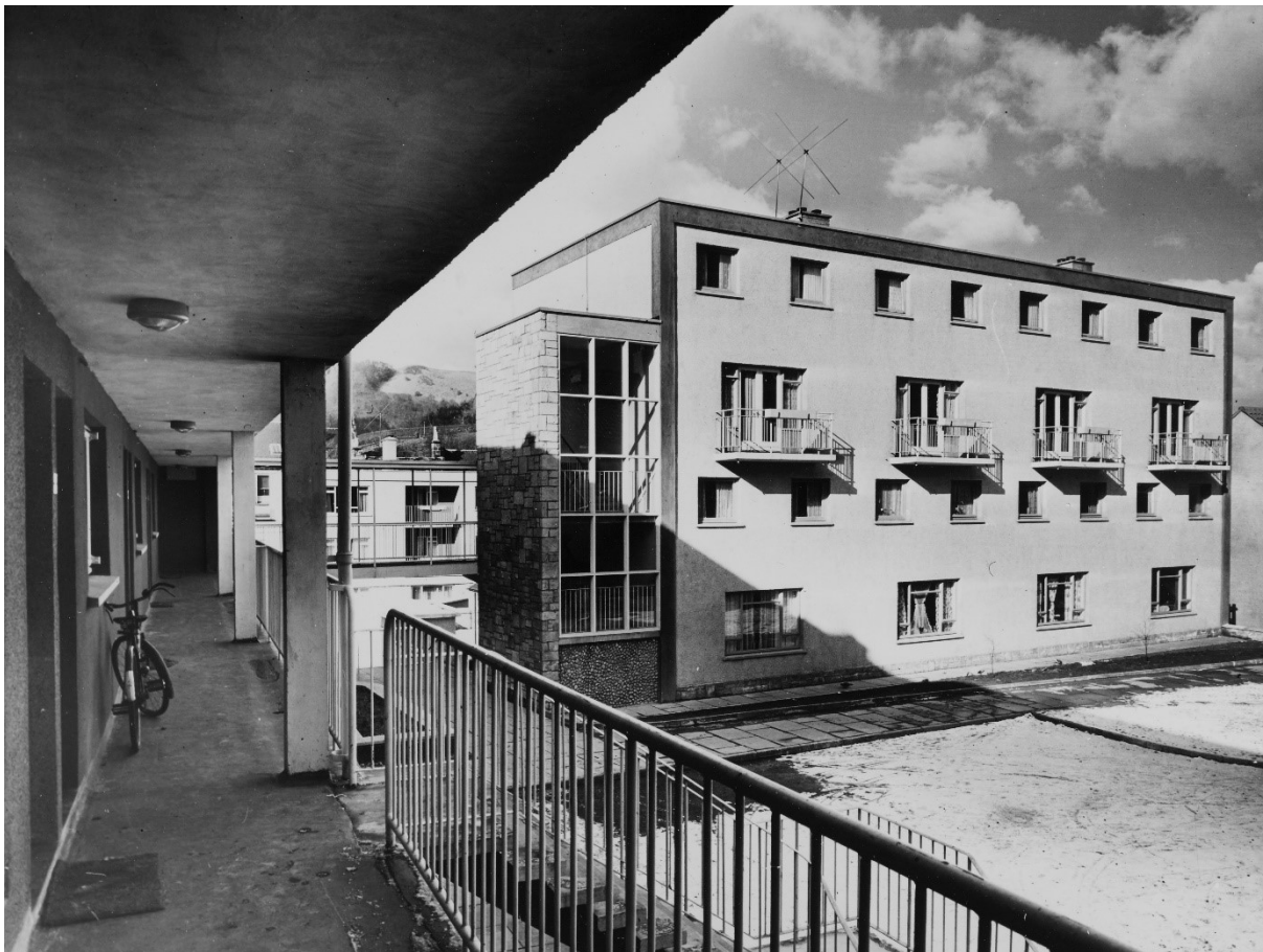
Figure 6.20. Glazed stairwells were used throughout the Burntisland and Dysart Developments. This example at Burntisland's Somerville Street/ High Street adds a sense of verticality to an otherwise horizontal building.
