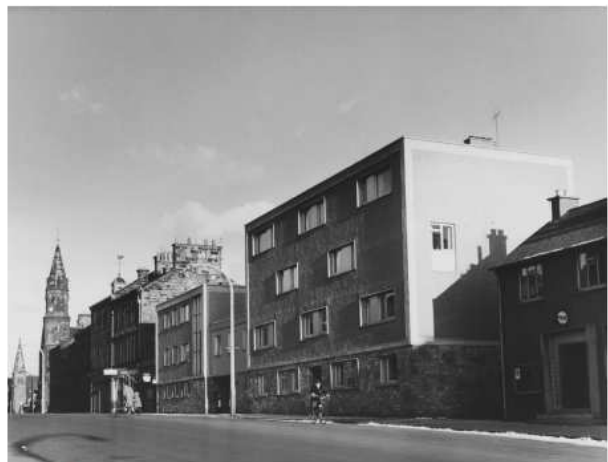
The High Street facing blocks
