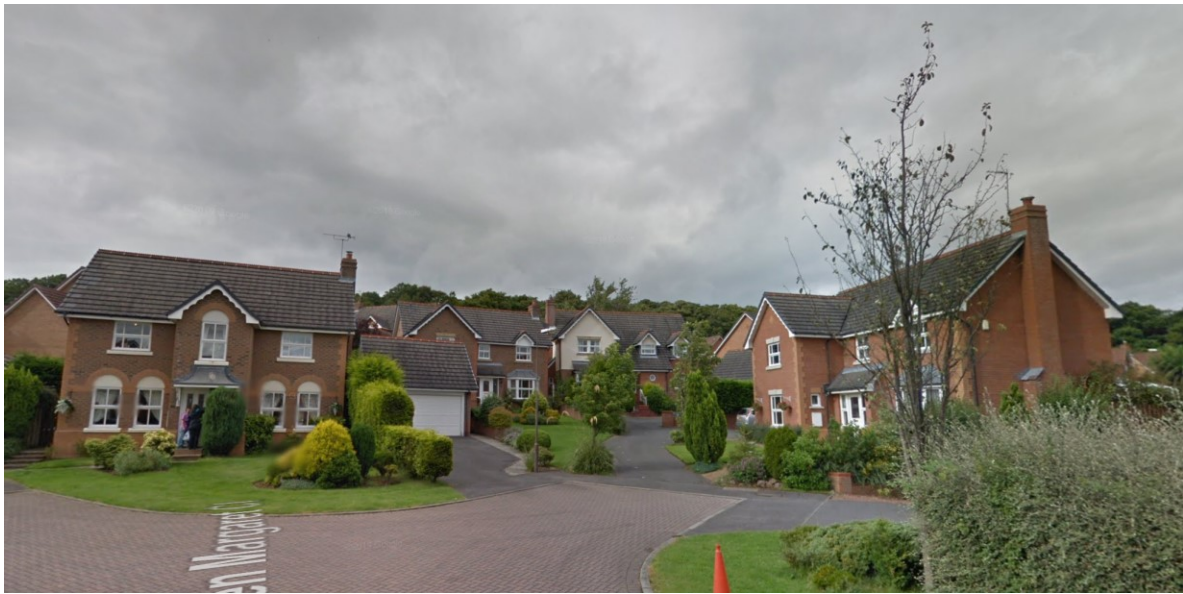
Figure C.5. These 1994 houses by Bryant Homes at Queen Margaret Close in the Buckstone Area of Edinburgh were criticised for their Victorian and English appearance.
