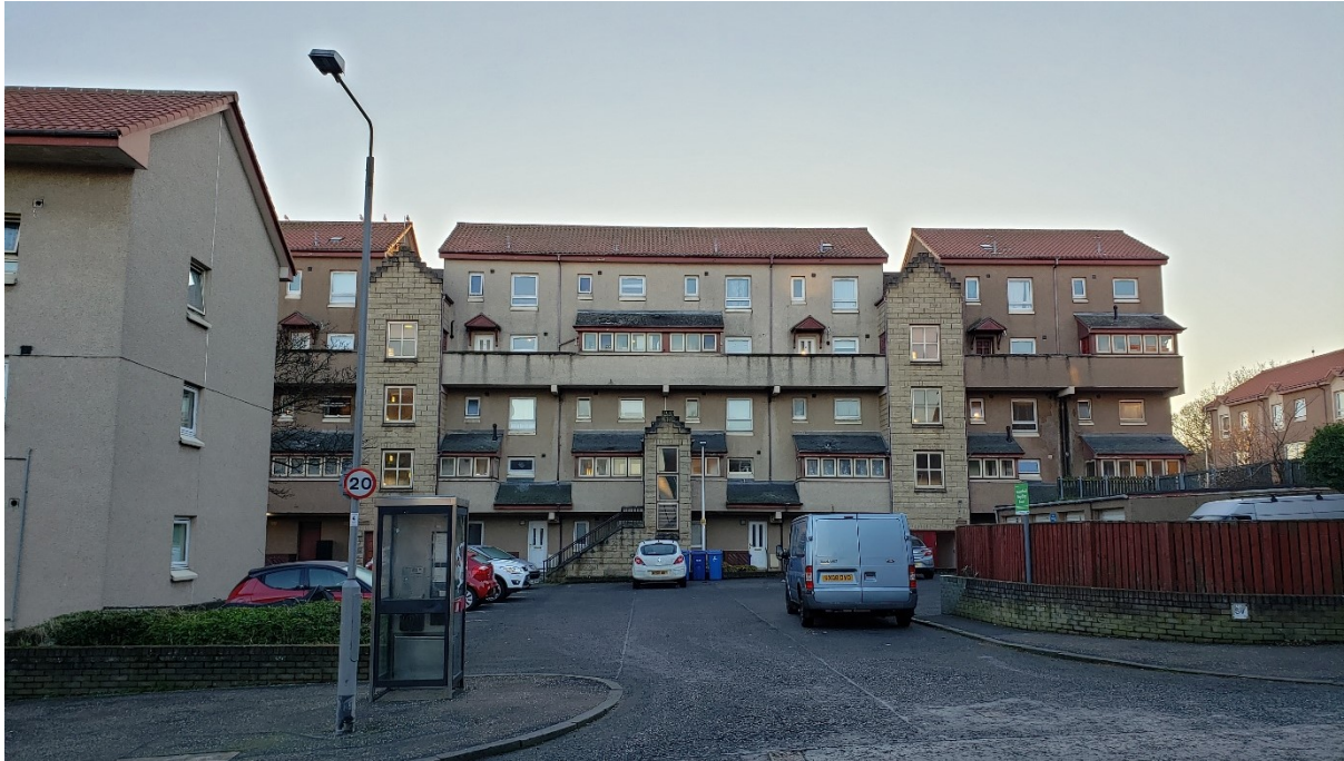
Figure C.11. Dysart's Phase 2, Block 5 received a dramatic redevelopment in 1997, with a pitched roof added, the access ramp removed, and crow stepped stair towers and canopies attached.
