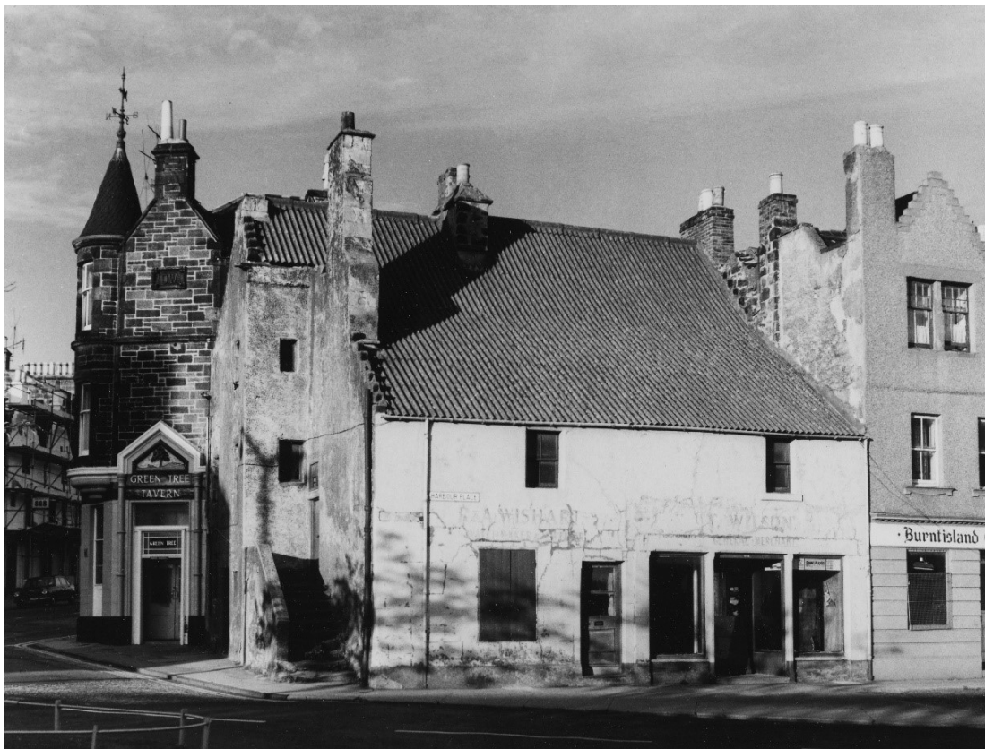
Figure 4.49. Image showing 1-2 Harbour Place prior to reconstruction. The photograph was likely taken shortly before work began in 1974.
