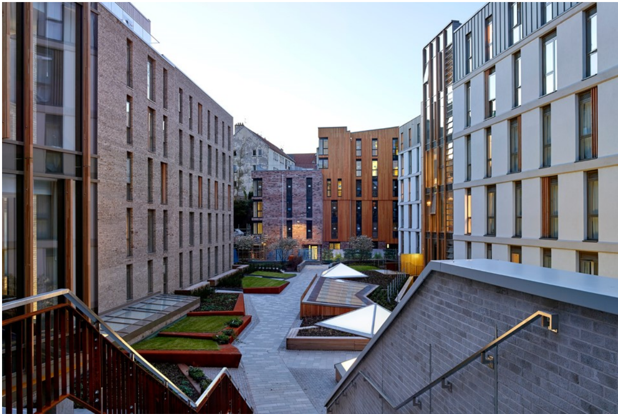
Figure 7.43. JM Architects' University of Edinburgh Accommodation and Outreach Centre, 2016.
