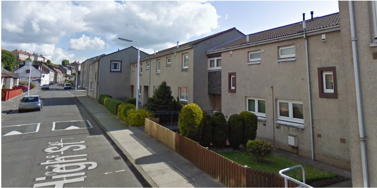
Figure 6.25. This example of Wheeler & Sproson’s more traditional terraced housing design can be seen here in Dysart’s Phase 3 – Part 2, but also in Burntisland’s Somerville Street/ High Street. Though there are distinct differences between these two examples, the blocks were generally topped with pitched pantile roofs and benefit from front and rear garden areas.
