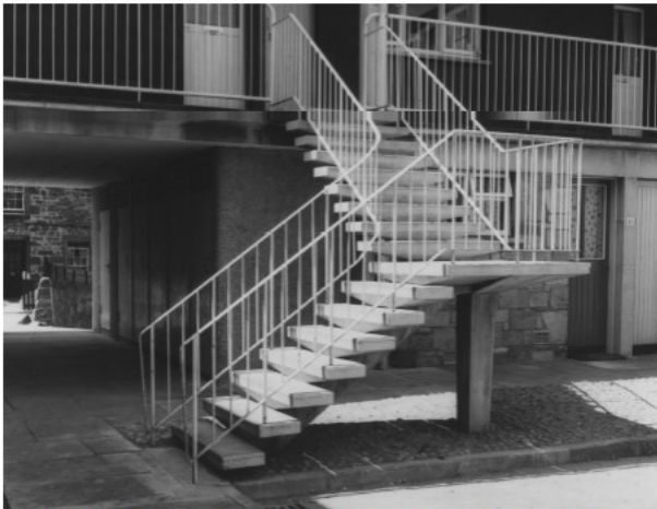
A modern concrete external stair was used in contrast with the traditional stone and harl behind at Somerville Street, Burntisland.
