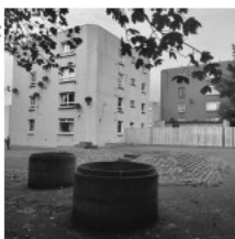
13) West Leven Street Redevelopment Phase 2 Dates: 1972—1973
