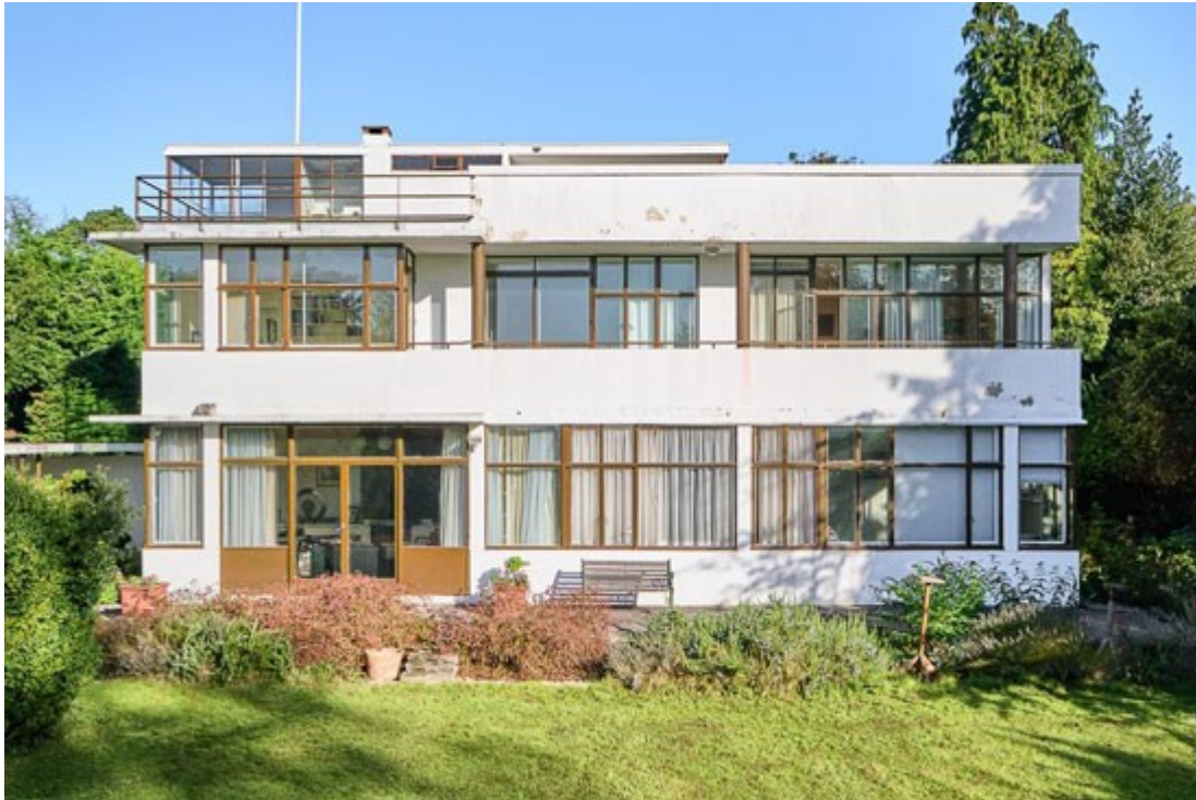
Figure 6.26. The horizontally emphasised Concrete House in Bristol by Connel, Ward & Lucas, 1934.
