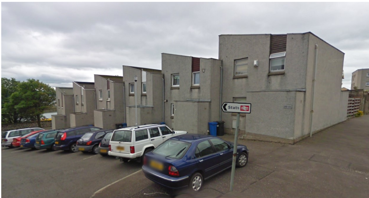
Figure 6.24. Mono-pitch terraced housing at the West Leven Street, Phase 2 development in Burntisland. These houses are almost identical in design to those in the 'unknown' phase on Somerville Street.
