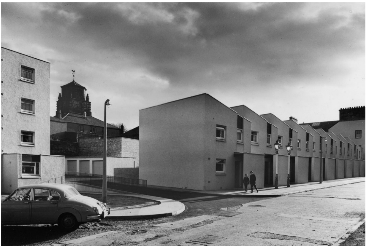
Figure 4.33. Photograph of the 9 terraced houses of the unnamed development, undated.
