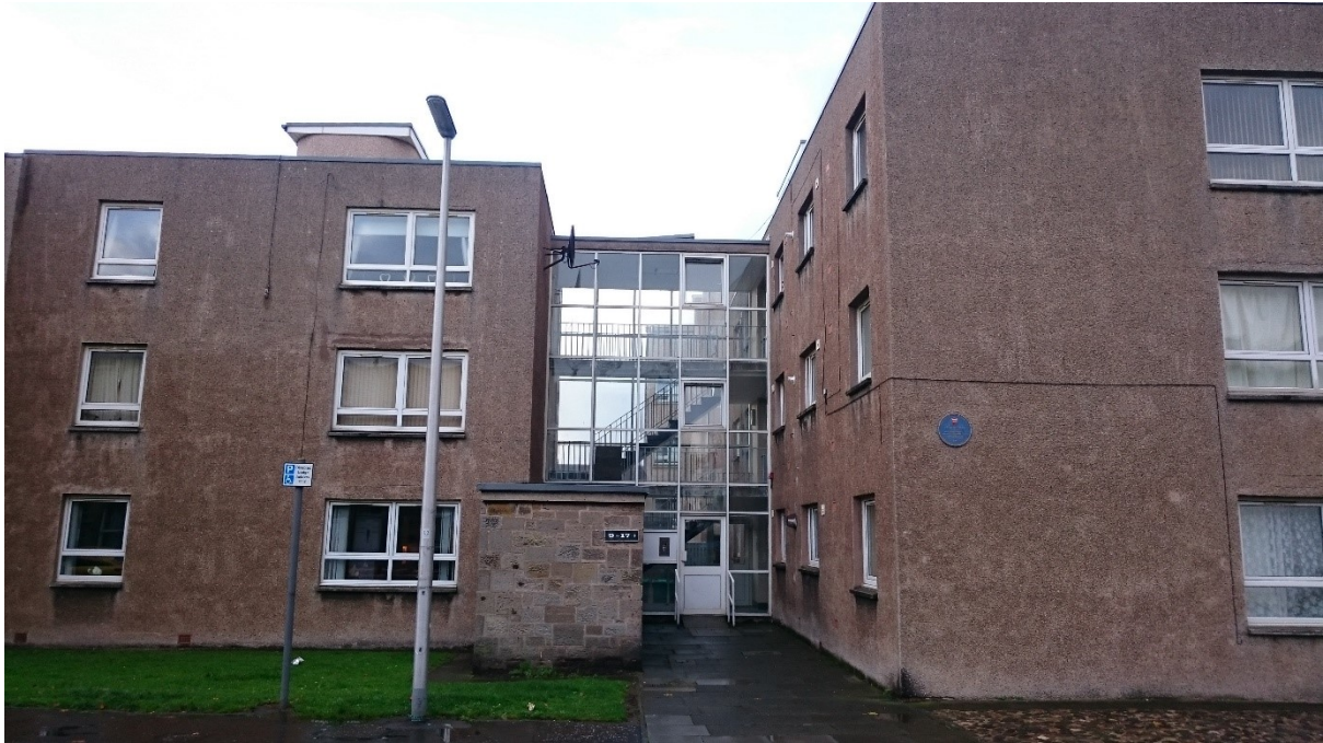
Figure 6.22. The Somerville Street Phase 2 development consists of two blocks of tenements connected and accessed through a central glazed stairwell.
