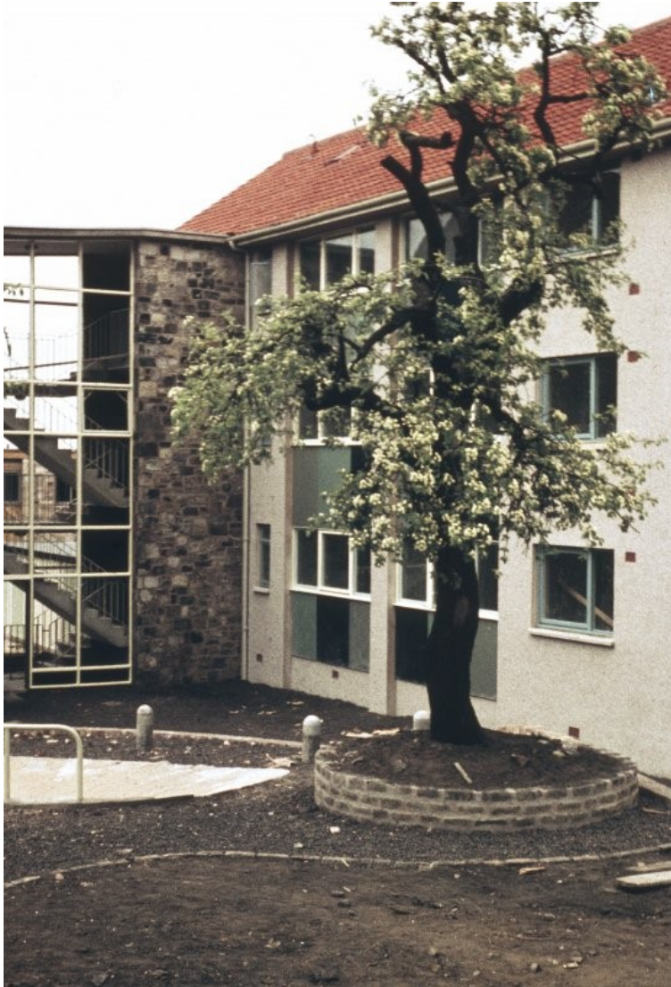
Figure 6.13. The only tree standing on the Dysart Phase 1 site when work began was this pear tree. Wheeler & Sproson designed Block A around the tree to protect it. Sadly, the tree has since been lost.
