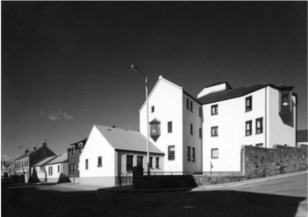
Figure 7.7. Baxter, Clark & Paul's 1977 Harbourlea sheltered housing in Anstruther made use of timber, steelwork and harling to blend in with surrounding buildings.
