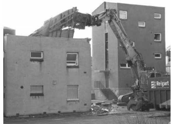
Image of the demolition of part of Dysart Redevelopment: Phase 2 in 2008.
