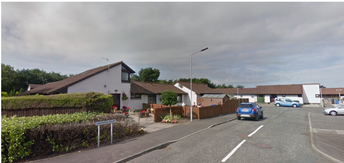
Figure C.3. The multi-award-winning Bryce Knox Court in Irvine by Roan Rutherford for the Irvine New Town Development Corporation follows many of the design concepts seen in architecture by the 1950s Modern-Vernacular architects, such as the use of pantiles and mono-pitch roofing.
