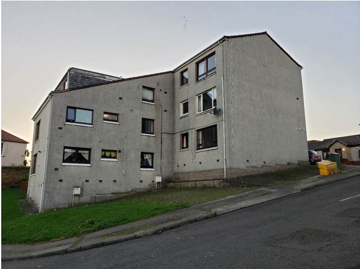
Figure 5.46. Dysart Phase 3 – Part 2, Block 10 taken November 2020.
