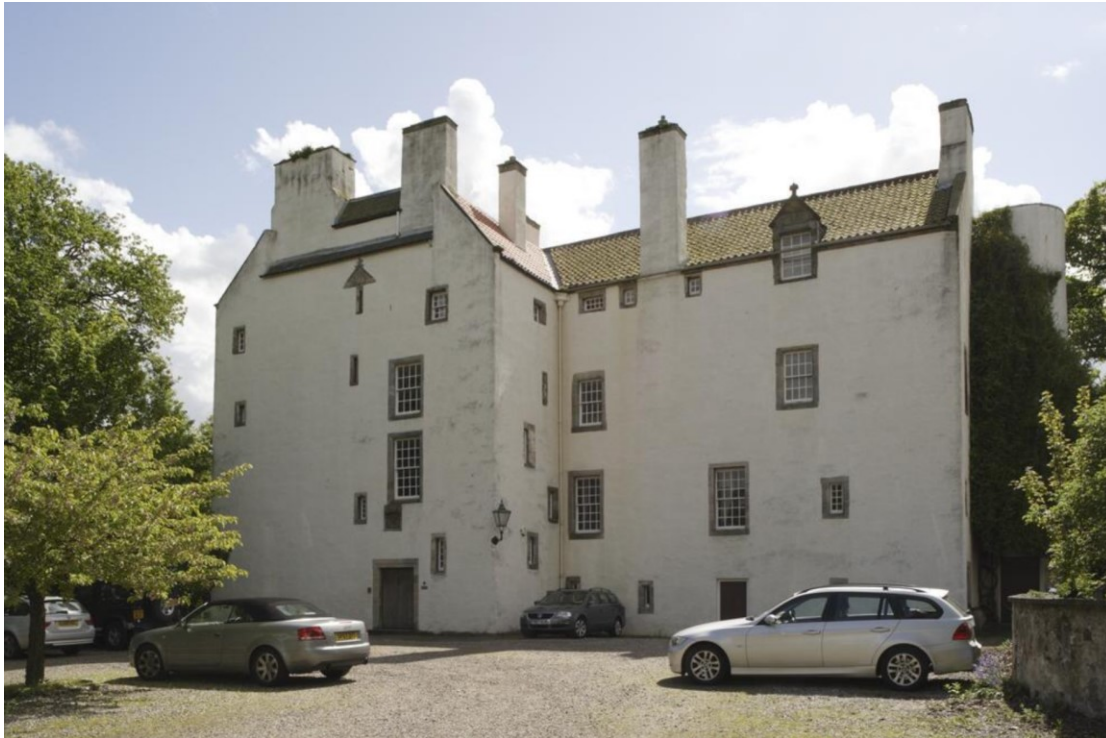
Figure 7.13. Rossend Castle was restored by Wheeler & Sproson in 1970 for the Links Housing Association.
