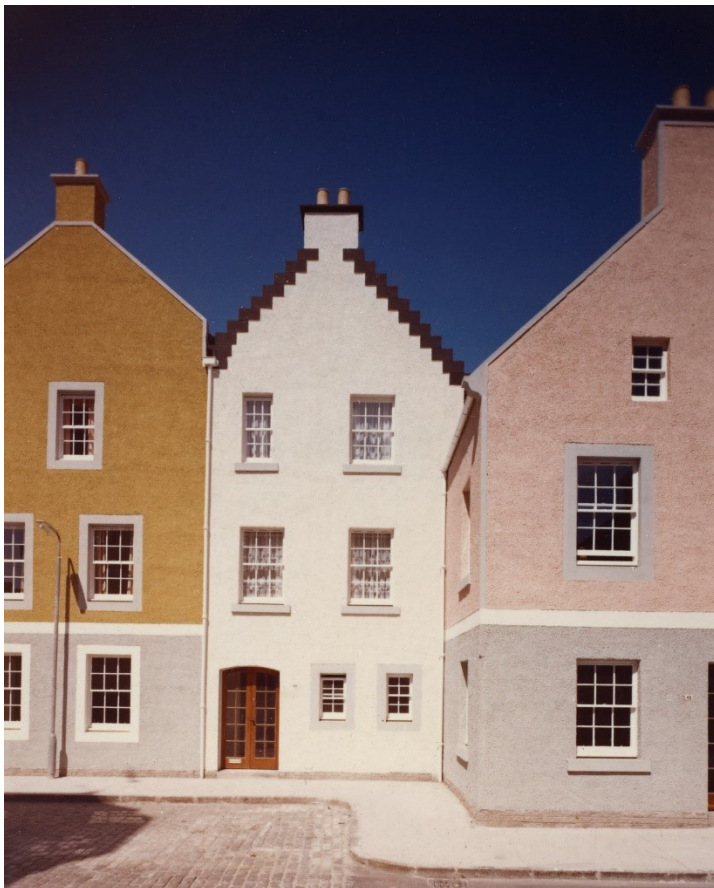
Figure 5.55. Image of 43-67 High Street (Job 514) post-completion, showing the bright use of colour adopted by Wheeler & Sproson for the reconstructed buildings.
