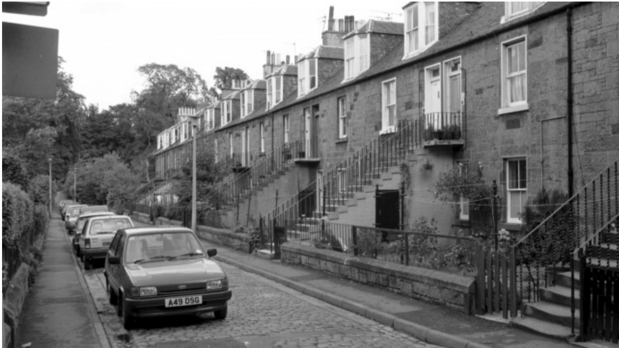
Figure C.8. Edinburgh's Stockbridge Colonies circa 1988, demonstrating the external stair access to the upper flats.
