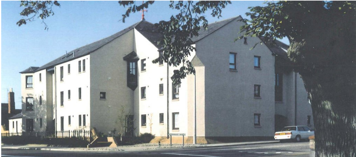
Figure C.2. Doward Gardens Montrose, by Baxter, Clark & Paul was a finalist of the 1994 World Habitat Awards, demonstrating its internationally recognised significance as sheltered housing.
