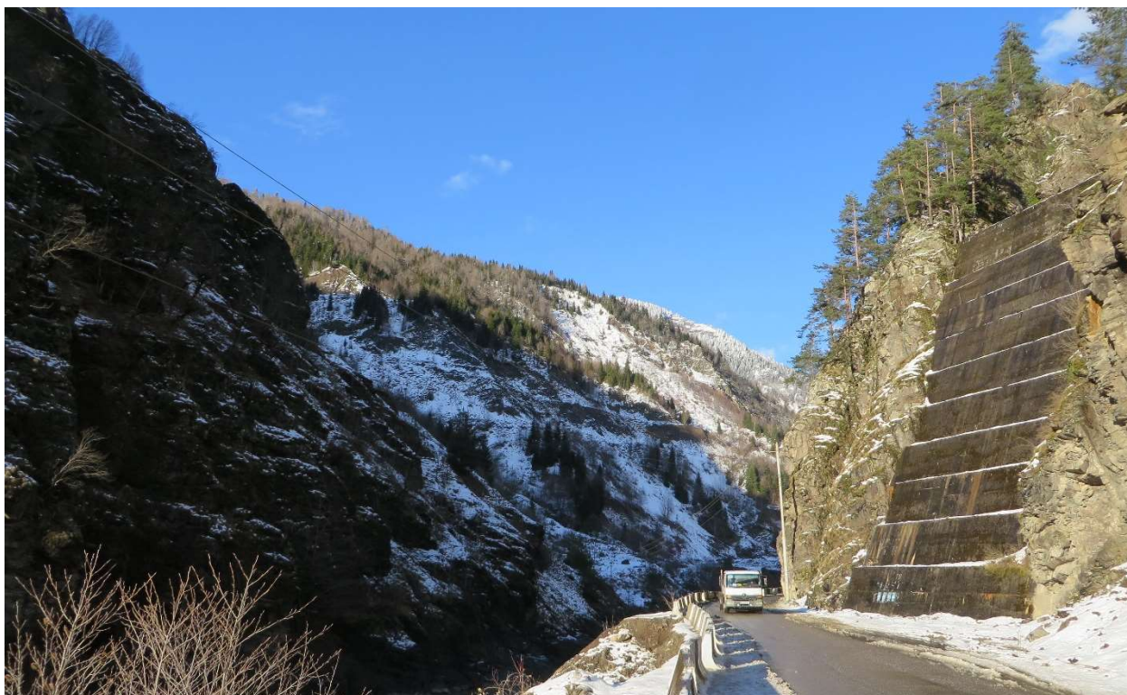
Figure 2.9: Unfinished beginnings of Khudoni HPP alongside the road into Svaneti
