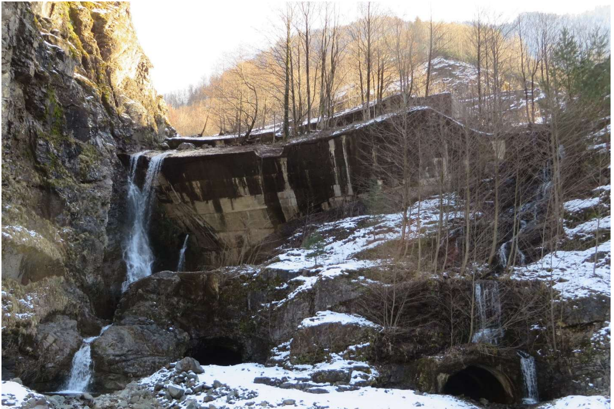
Figure 2.8: Unfinished beginnings of Khudoni HPP alongside the road into Svaneti
