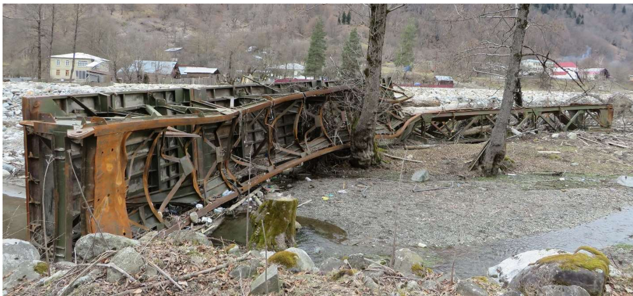
Figure 6.6: The old bridge from Chuberi, still lying where it was carried to by flooding in summer 2018 Source: Photo by the author, February 2019.
