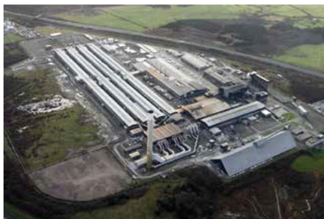
FIGURE 2: Anglesey Aluminium Plant prior to closure (Crown Copyright: Royal Commission on the Ancient and Historical Monuments of Wales)
