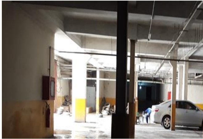
Figure 10. Using natural daylight to illuminate the basement parking area
