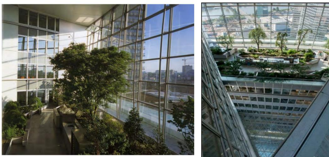
Figure 16. Passive Solar: The sky gardens and offices are surrounded by large glass facades that allow for direct and indirect solar benefit for the majority of the year when heating is needed. To avoid overheating, internal shading mechanisms and ventilation systems are used. 27
