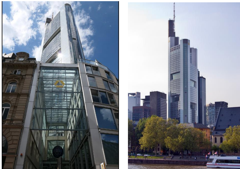
Figure. 11 and 12. Exterior View of Tower C 27
