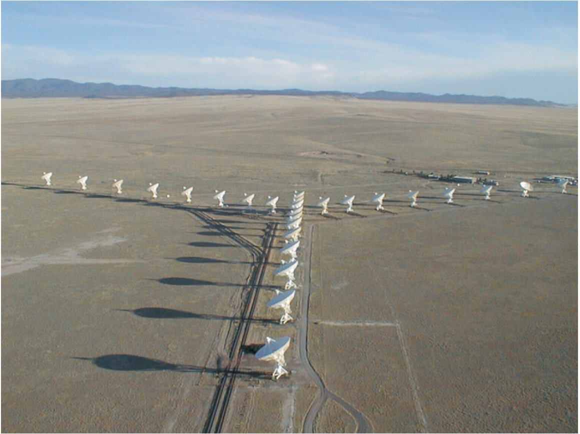
Figure 1.11. The Karl G. Jansky Very Large Array, located around 80 km (50 miles) west of Socorro in New Mexico. The array is distinctive for its Y-shape configuration of antennas. Image credit: NRAO.
