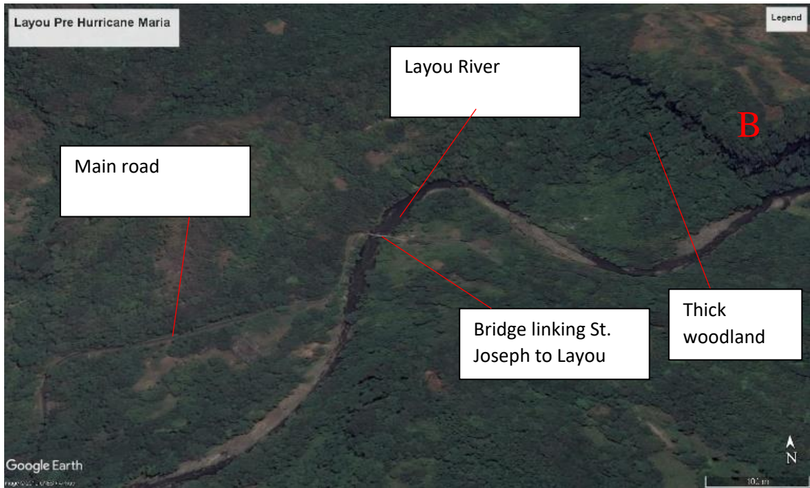
Figure 5.3 B: Google Earth images before the Hurricane Maria event for Layout (Dominica)
