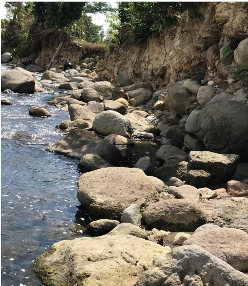
Figure 5.15: Delice River field photograph showing lateral deposition of boulders (0.5-3.4 m in diameter) from the riverbank failure caused by excessive force of the flow and hydraulic toe erosion undercutting the river-bank during Hurricane Maria. River flows from right to left from the viewer.
