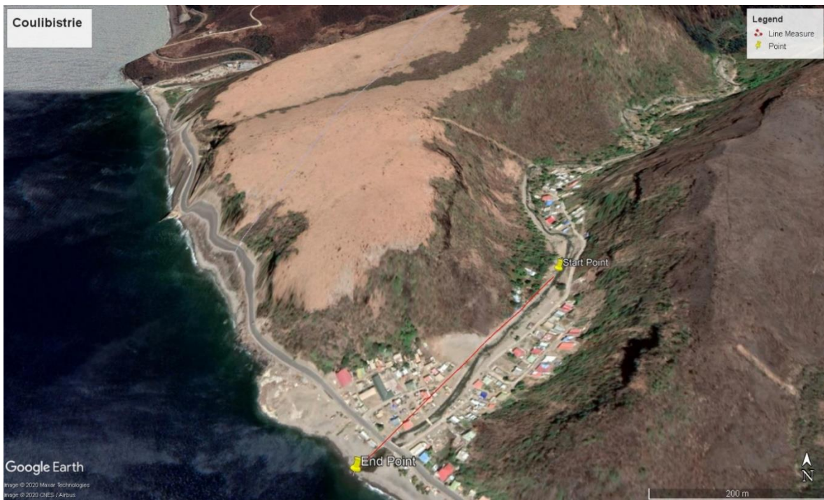
Figure 3.23: Google Earth Map of Coulibistrie area where a drone survey was conducted.
