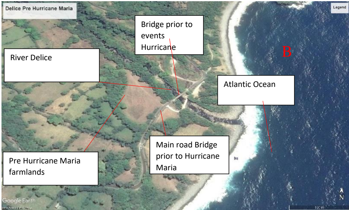
Figure 5.2 B: Pre-Hurricane Maria Google Earth images for Delice (Dominica)
