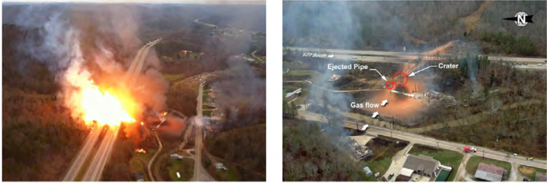
Figure 1.1: The accident scene of pipeline rupture [1].
