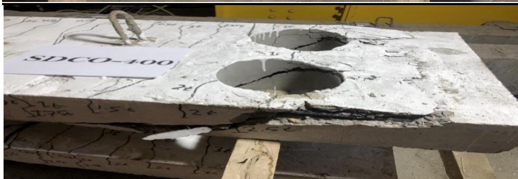
Figure 7. Cracks of SDCO-400 slab.
