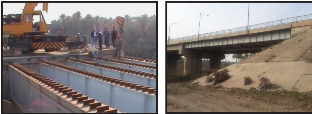
Figure 12. Al SABIYA Bridge.
