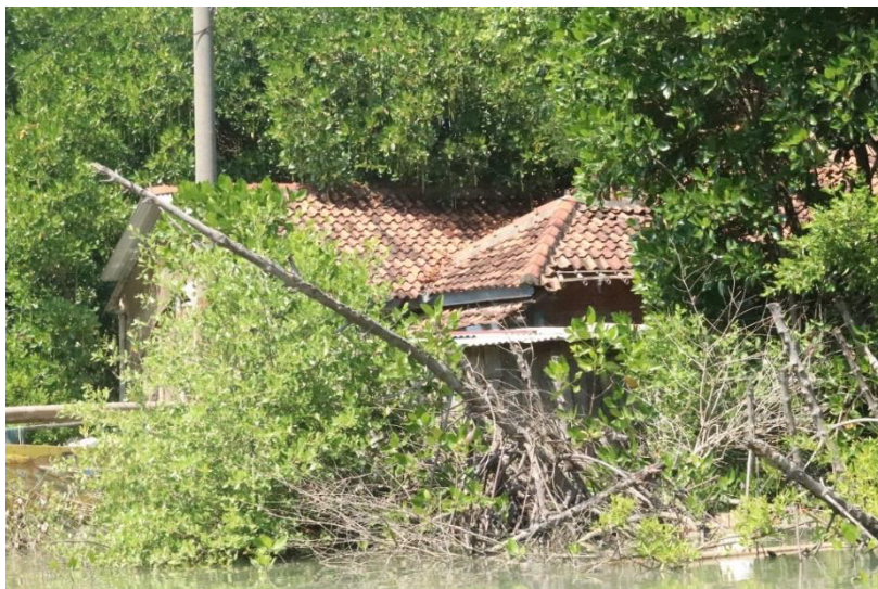
Fig. 1. One of the houses left by the occupants because of the overflow of tidal water.
