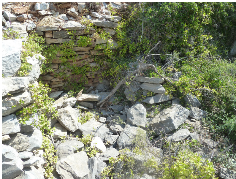
Fig. 4. A rectangular chamber at the lowest part of the path towards “Karavi” quarry.
