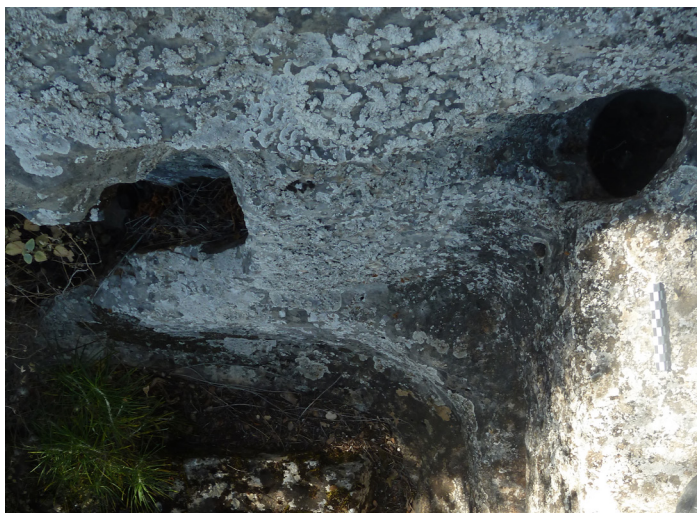
Fig. 17. Holes for the secure fastening of ropes used for the transportation of the blocks in the quarry.
