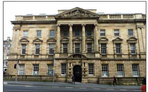
Midlothian County Buildings, King George IV Bridge, Edinburgh, Geological Survey housed here 1879-1906 (K.J. Edwards)
