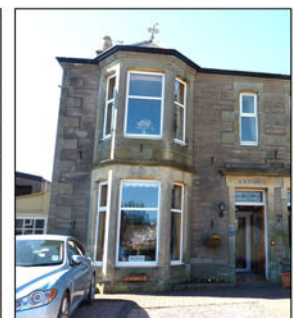
5 Pitcullen Crescent, Perth 1886-90 (K.J. Edwards)
