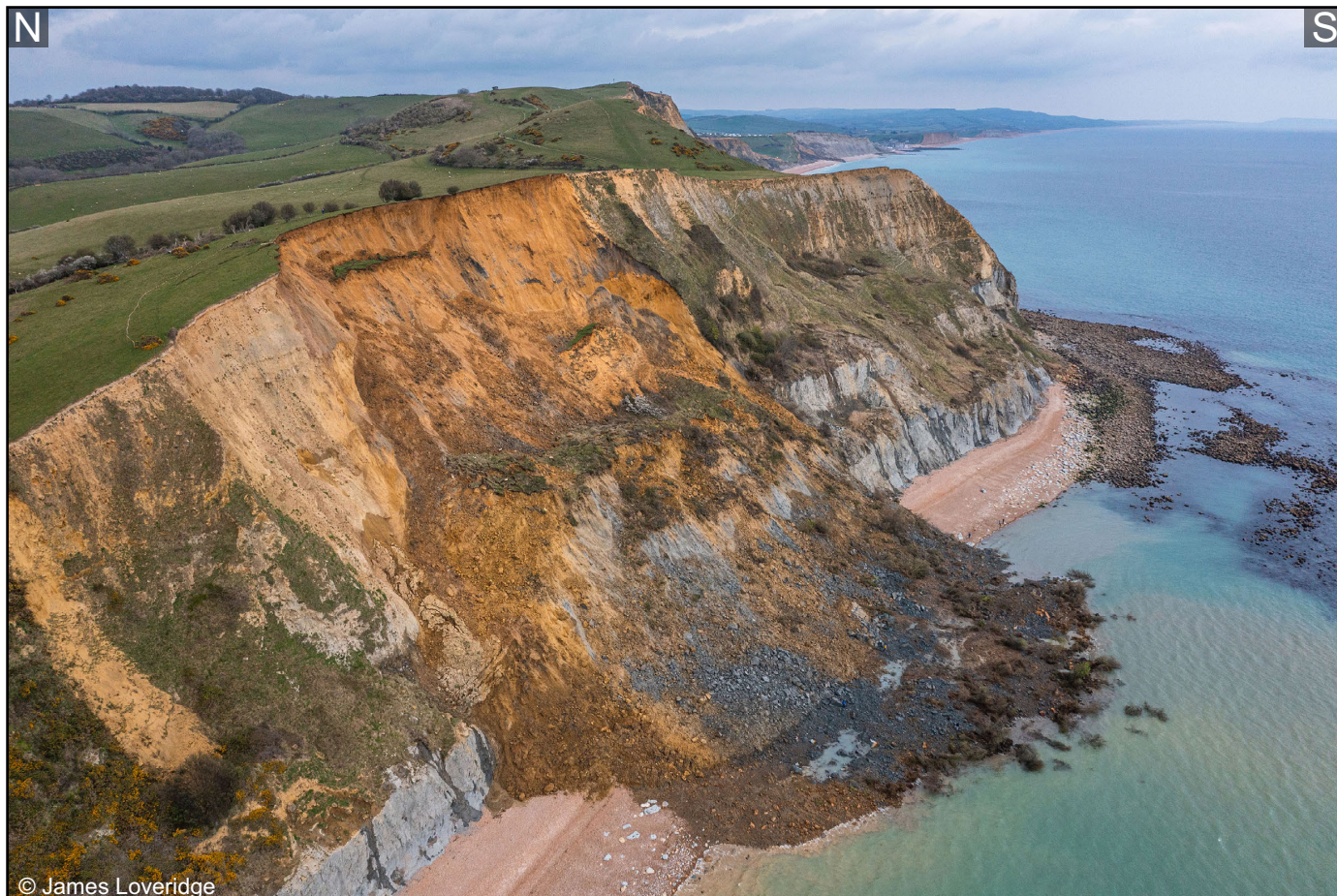
Figure 4: Image of the largest rockfall (greater than 4,000 tonnes of debris) in 60 years, in the UK. The collapse occurred along the Jurassic Coast, a UNESCO World Heritage Site. These important, cliff-forming outcrops are highly susceptible to collapse, deterioration, and destruction. Cliff is approximately 85 m tall. Photo courtesy of James Loveridge ( https://www.jamesloveridgephotography.co.uk/the-jurassic-coasts-biggest-cliff-fall-in-60-years/ , April 2021).
