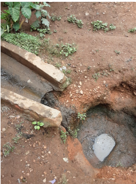
Figure 9: Urine storage in a pit with no floor and cover: a lot of the urine nitrogen is lost through leaching and volatilization of ammonia.
