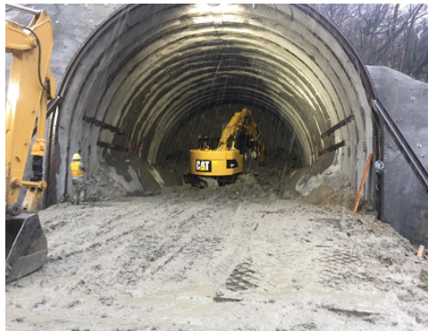
Photo of tunnel excavation
