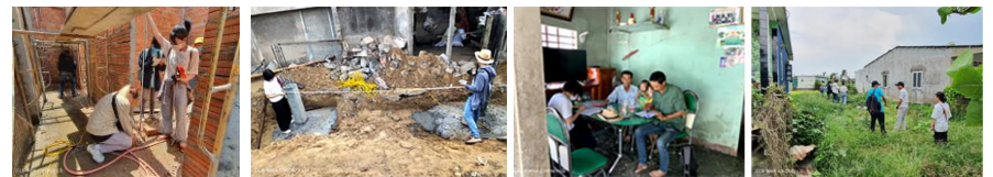
Fig.4. field surveys and construction process supervision
