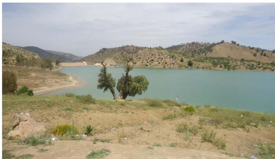
Figure 3. Photo of Koudiet Rosfa Dam
