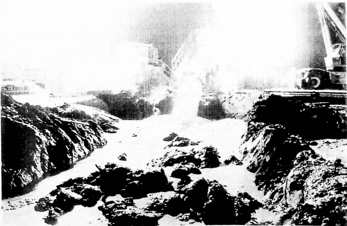
Figure 5.13 Pipe pull through completed. The pipeline emerges having been pulled through the a directionally drilled pilot hole. Source: VneshTruboProvodStroy et al. , 1994.
