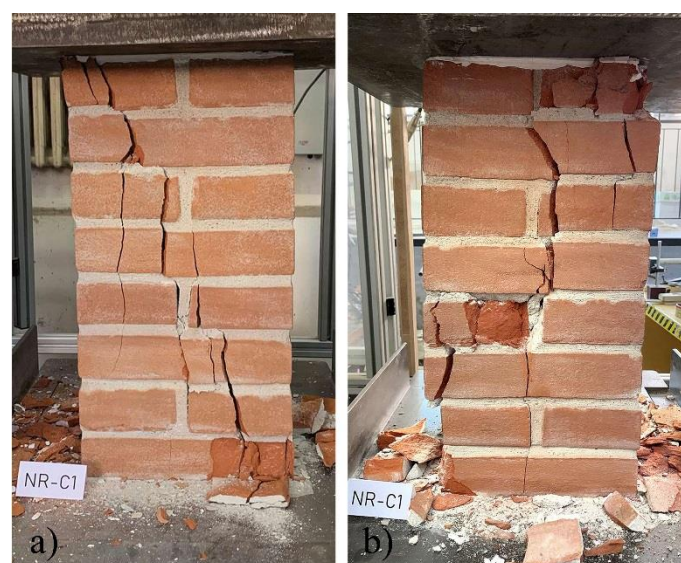
Figure 9. Reference failure mode of unreinforced masonry columns (NR-C1 specimen): (a) front and (b) back sides.
