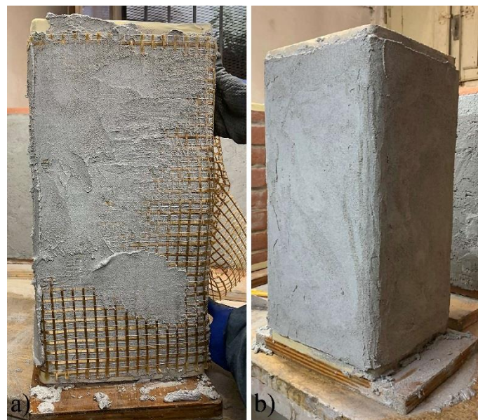
Figure 8. Columns strengthened with the FRLM composite. (a) Execution of the first layer of matrix and positioning of the textile. (b) Specimen completed with the second layer of matrix.
