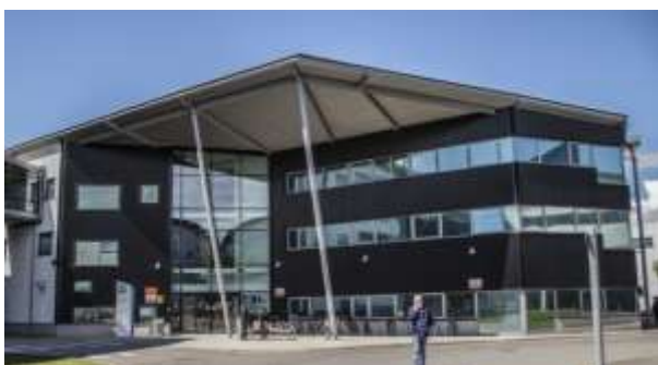
Figure 3: External southeast elevation of the building demonstrating the metal cladding and fenestrations.
