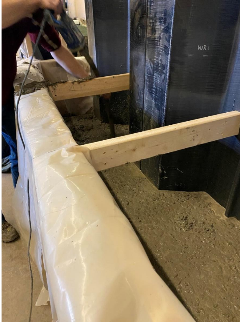
Figure 4. 5:Concrete Poured Around Specimen
