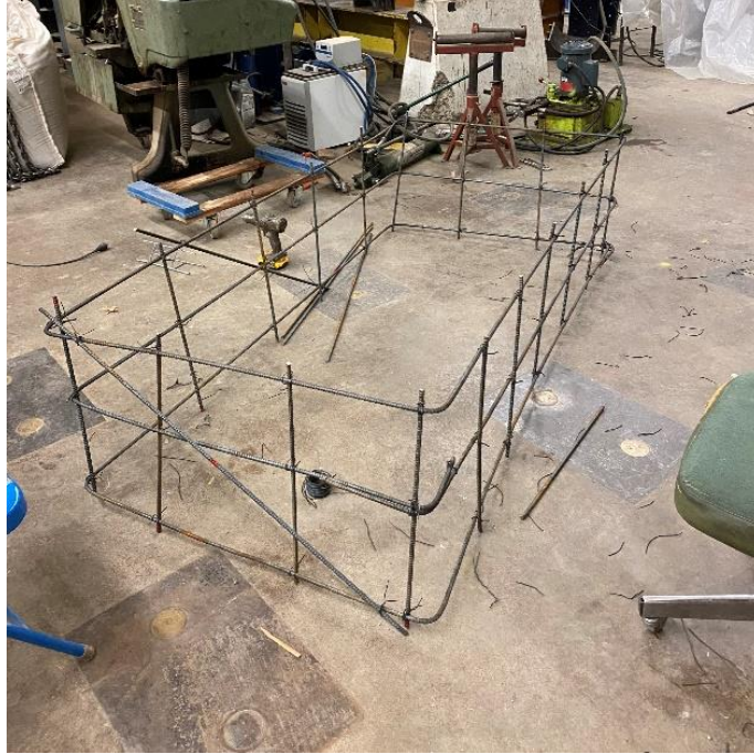
Figure 4. 9:Concrete Reinforcement Structure
