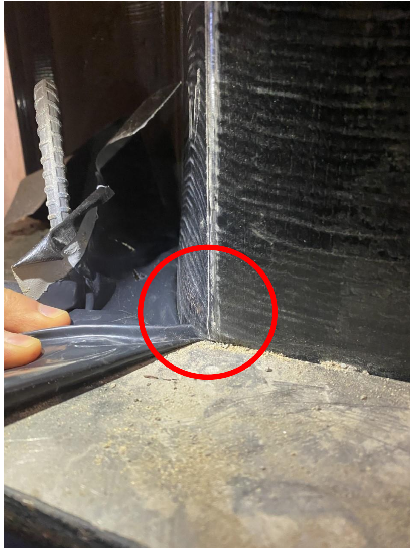
Figure 4. 16: Buckling about Weak Axis
