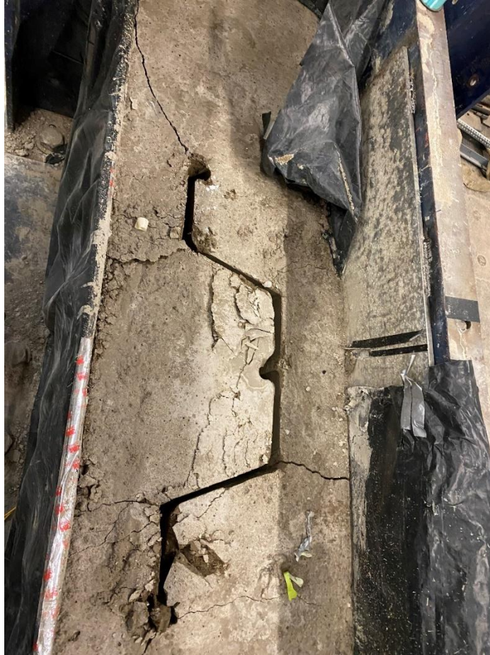
Figure 5. 19:Embedment Material Post-Test
