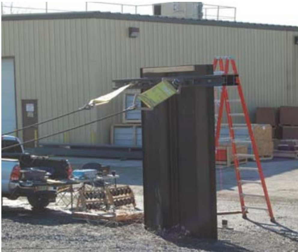
Figure 3. 1: Field Sheet Pile Test
