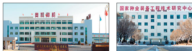
Fig. 2. National Engineering Technology Research Center of Seed Processing Equipment
