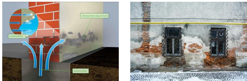
Fig. 4 Capillary moisture, initiator and cause of damage occurring on the walls and foundations [7]
