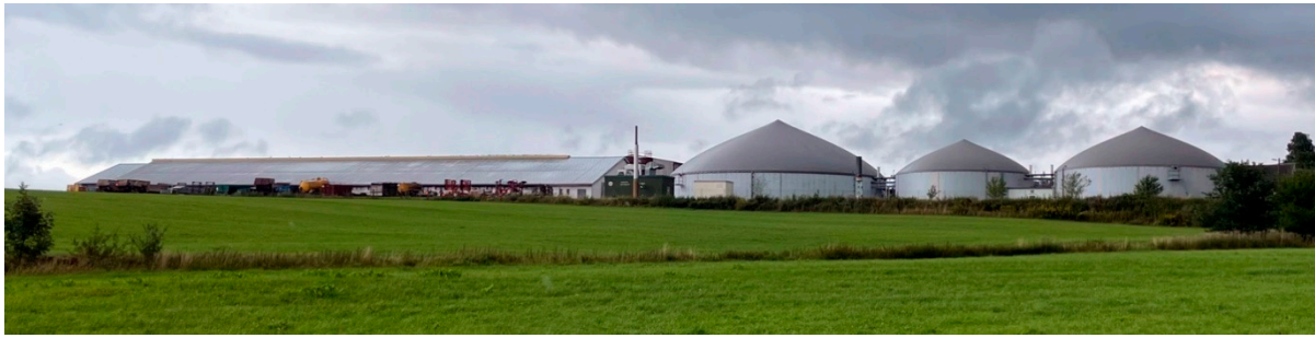
Figure 3. Biogas station on part of the area of a former collective farm. Image by Tomáš Krejčí (Chlumec near Dačice, the Czech Republic, 4 June 2021).
