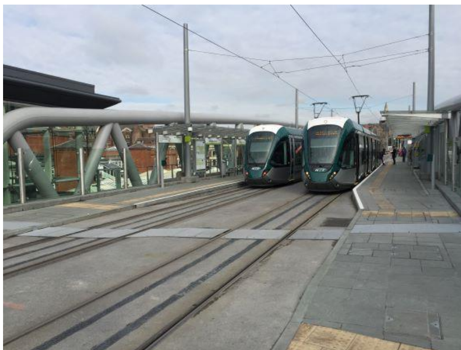
Figure 6-5: Trams at the new Nottingham Station tram stop on the Overbridge during testing at handover
