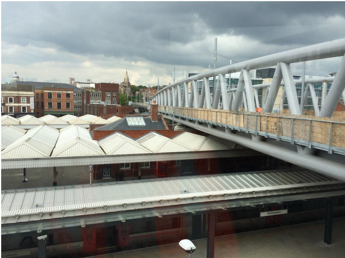
Figure 5-1: View of Nottingham Station with the recently installed tram bridge oversailing the platforms
