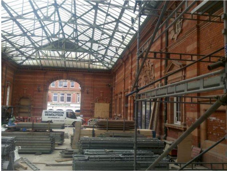
Figure 5-2: Nottingham Station Porte-Cochere during Construction
