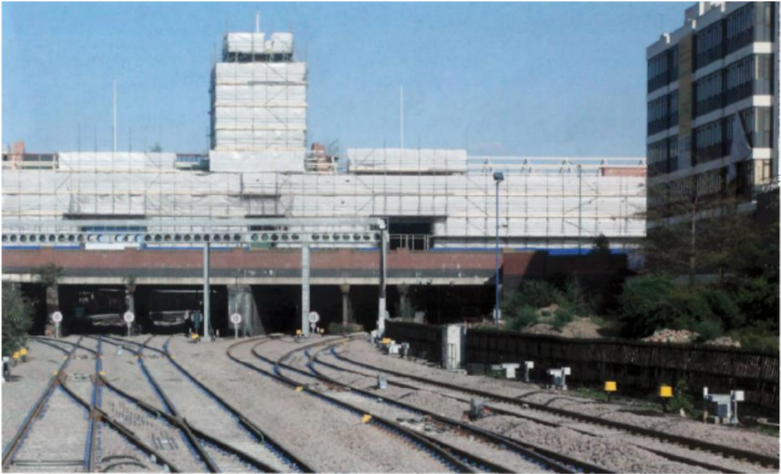
Figure 6-7: Approach to Nottingham Station during the refurbishment passing under Carrington Road
