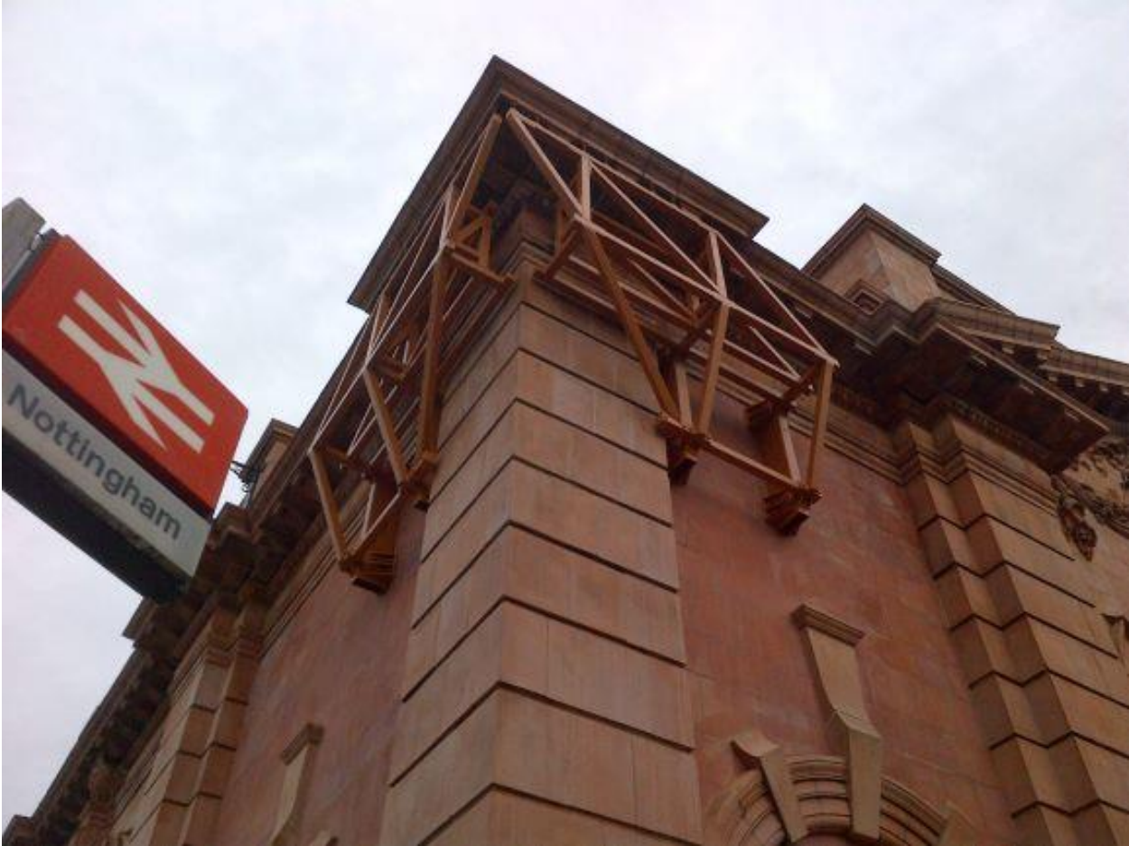
Figure 5-6: Refurbished Terracotta Façade of Nottingham Station with temporary corner bracing
