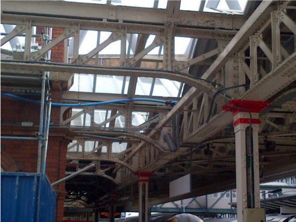
Figure 5-9: The reglazing of the platform canopies showing temporary cabling and containment.
