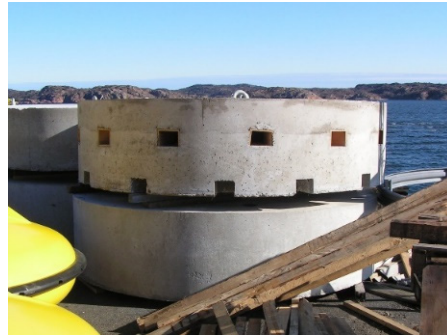
Figure 2. Two ecological foundations for environmental and ecological studies in the Lysekil wave power park research site. Upper ecological foundations include manufactured holes for increased complexity.
