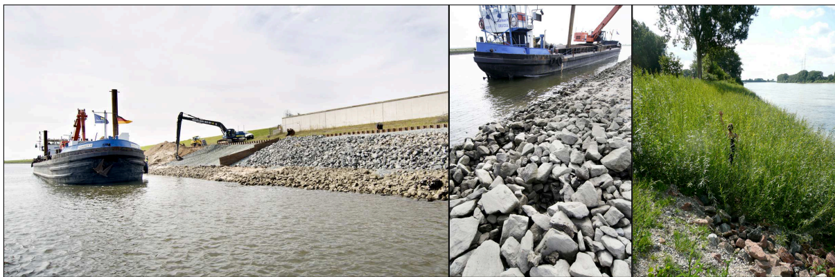
Figure 1.1: Common bank protections at inland waterways (Photos: BAWArchiv).
