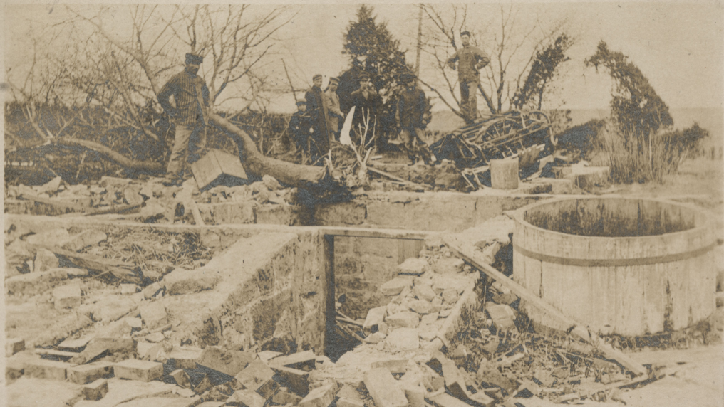
9104A. CELLAR OF VANBUSKIRK WHERE 5 LIVES WERE SAVED HIWATHA MANS.
