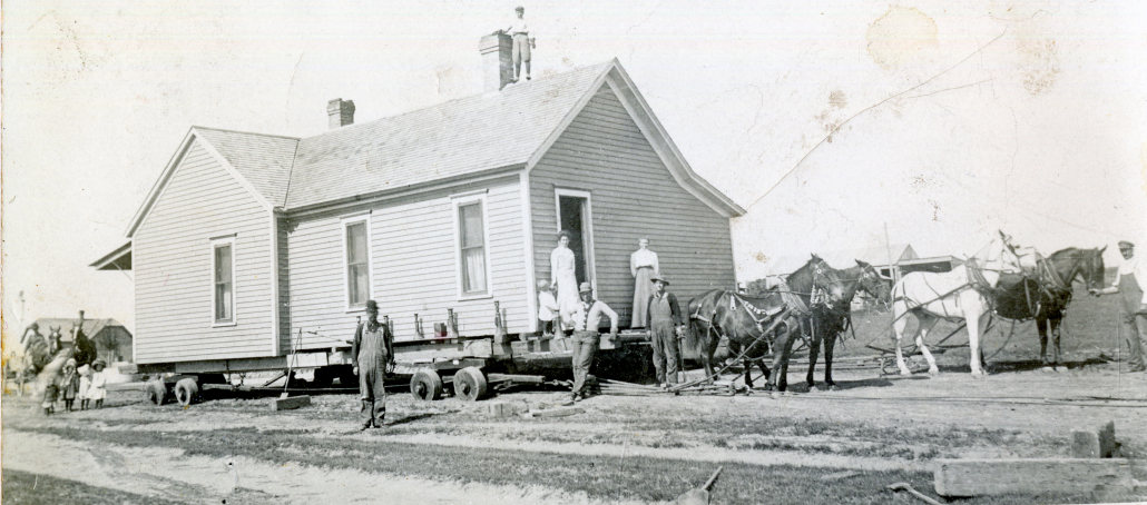
Moving Roll Brock Residence, Jennings Kans. GEO. W. JACKSON (HOUSE MOVER) OBERLIN KANS.
