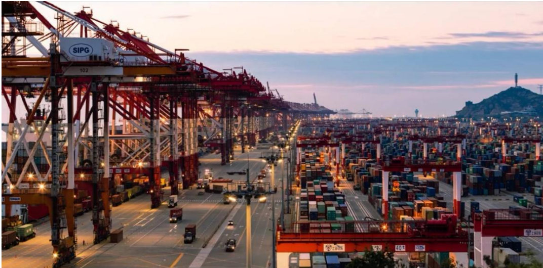
Fig 4 Yangshan Phase IV fully automated container terminal
