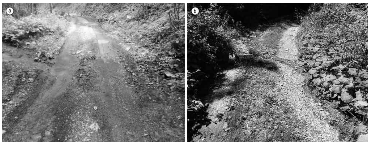
Slika 8a i 8b. Otjecanje vode preko kolnika Fig. 8a and 8b Water runoff over a roadway
