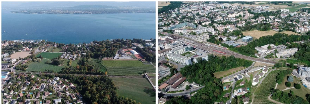
Fig. 2. Aerial views of sectors Bois-Bougy (left) and Nyon-Prangins (right)
