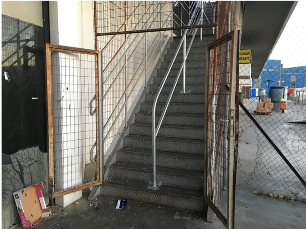
Figure 3. Elliniko Arrivals Refugee Site entrance access point. A. Paraskevopoulou, 2016.
