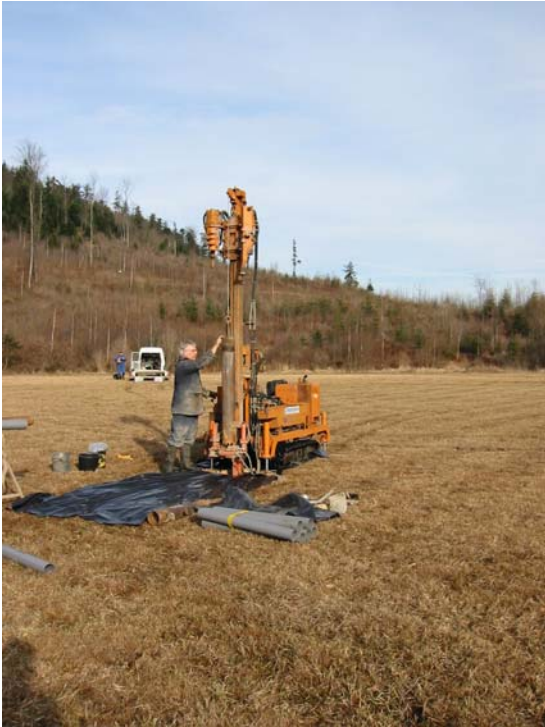
FIGURE 3.3.2 Picture of the Gasserplatz with the mechanical auger (March 2002).
