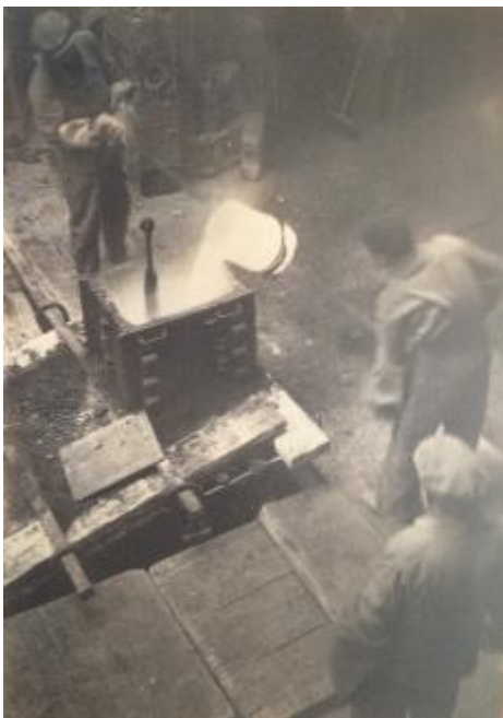
Fig. 4.49. Foundry men filling the runner box on top of a large mould in the Alexis Rudier foundry Paris (1934-36). Pulling the plug allowed the content of several crucibles to flow at once. (original photograph probably by C. Mitchell, from the Malvina Hoffman papers, Box 15.2, Special Collection Getty Research Institute, L.A.)
