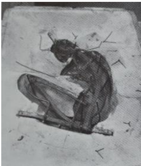
Fig. 4.32. Core armature inside the drag mould (from Kowalski & Weisner 1984, 20)
