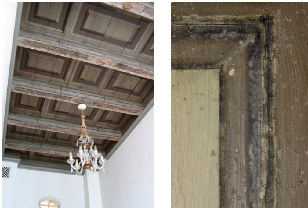
Fig. 4.4.1 Unknown artist(s), Painted ceiling with panel imitations (Johan de Witt House, The Hague, room 1.12), 1652-55, oil on panel ( left ) and dark shadows affected by whitening ( right detail )
