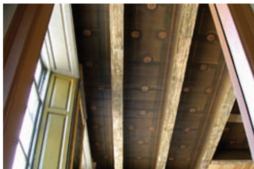
Fig. 0.5 Painted ceilings (1652-55) of the Johan de Witt House, The Hague. The panel imitations, originally applied in various green tones, now show uniform brown colors ( left ). Cross-section analyses revealed a brownish paint containing verdigris (copper green) and lead white that are slowly converting into metal soaps ( right ).
