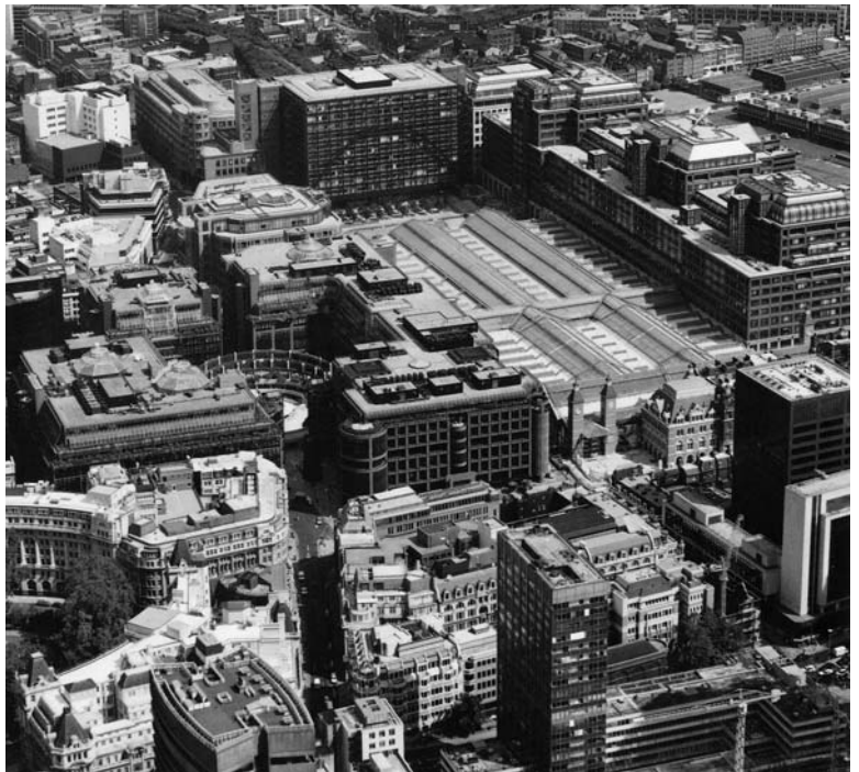
Figure 2. Broadgate, typifying the 'property capitalization' approach. (Source: Broadgate)
