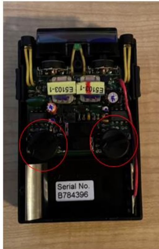
Figure 3.1: EMS unit control panel (photo by Pablo Valenzuela)
