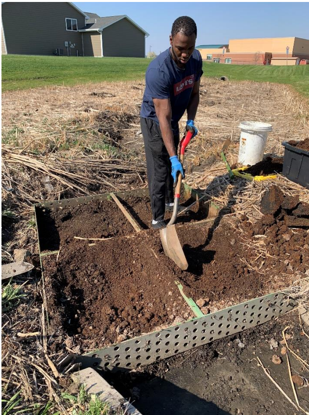
Figure 8. Process of adjusting the steel byproduct ratio for the pilot scale steel byproduct filter.
