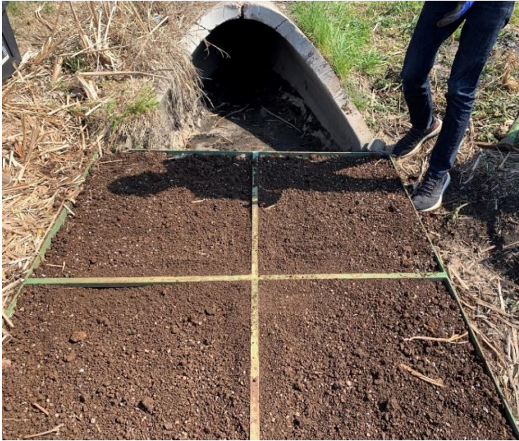
Figure 11. Pilot scale steel byproduct filter after ratio adjustment.
