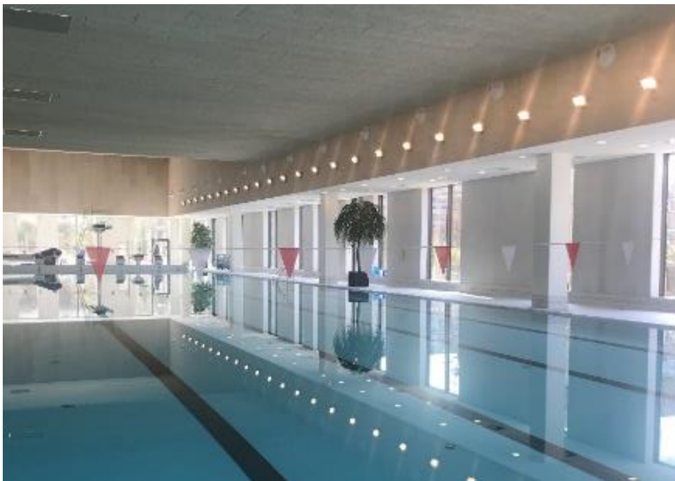
FIGUR 28. As built af 50 m bassinet. Kilde: BUILD/AAU.
