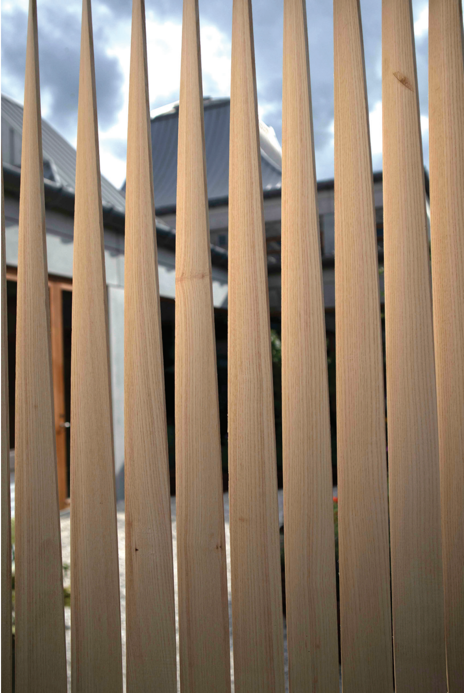
Figure 6.1. Physical demonstrator of the wood lamella facade. Exhibited in the Utzon Center, Aalborg, Denmark. Photo by Mads Brath Jensen.
