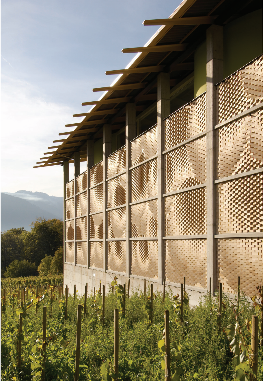
Figure 1.3. The robotic fabricated brick facade of the Gantenbeim Winery, 2006, Switzerland. Project by Bearth & Deplazes Architekten and Gramazio & Kohler. Photo by Ralph Feiner.
