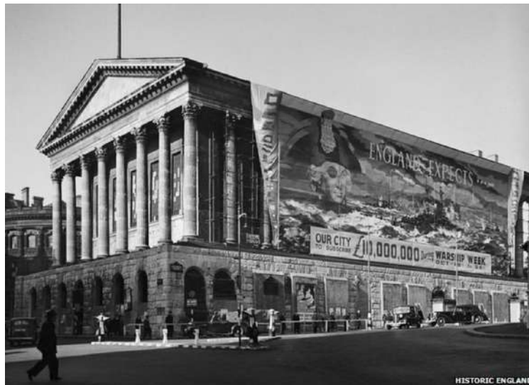
Fig. 1 - Birmingham Town Hall, Victoria Square, Birmingham 1941. George Bernard Mason (1896-1985), National Building Record. Source: https://www.bbc.com/news/in-pictures-33408095
