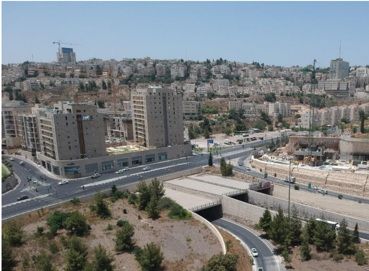
Figure 2. "Mordechai hill" interchange
