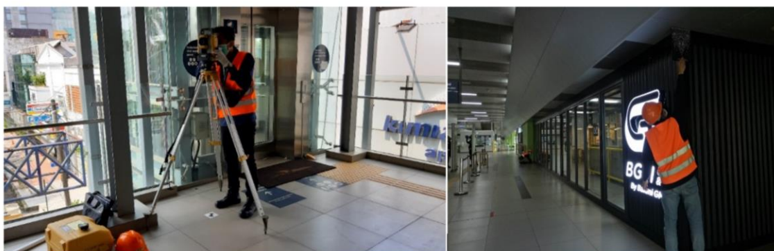
Fig. 10. Validation survey by using Total Station and distometer (Atunggal et al., 2020)
