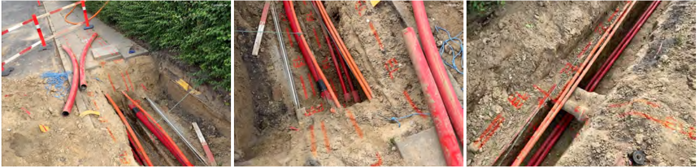
Fig. 15. Virtual utility markings overlaid onto real excavations. Because our algorithm is able to mark lines even during excavation works, it is possible to validate the accuracy of GIS data with respect to the actual physical location of utilities. Markings deviate by a few centimeters, in particular from soft cables, but the AR overlays successfully guide the daylighting.
