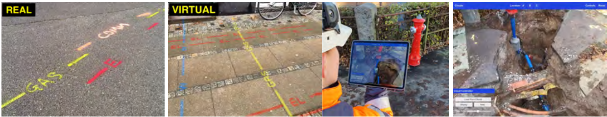
Fig. 1. Virtual utility marking and daylighting in comparison to physical counterparts: (left) physical spray markings on the street surface, (mid left) virtual utility marking of similar information in AR, (mid right) worker examining a virtual excavation in Aalborg (Denmark), (right) AR view with embedded 3D reconstruction of said excavation.
