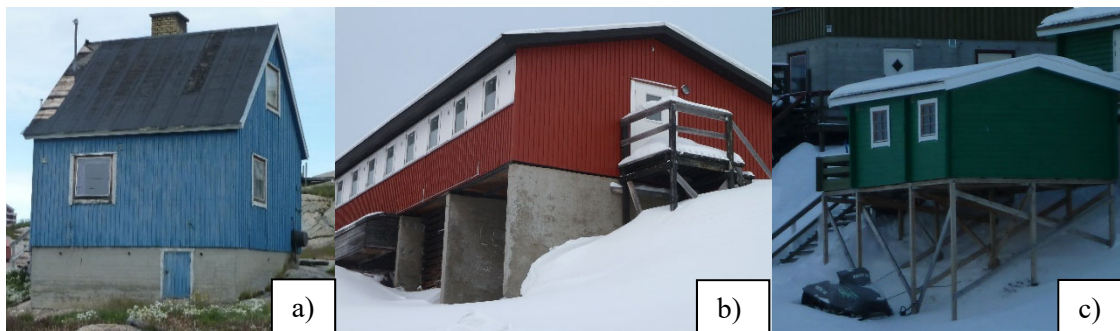
Figure 5. Different ways to support buildings in Greenland, a) a closed in-situ casted concrete construction with openings for ventilation, b) a partly open concrete construction, c) a wooden construction, leaving the floor construction fully exposed.
