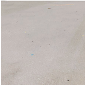
GROUND MATERIAL: Concrete
