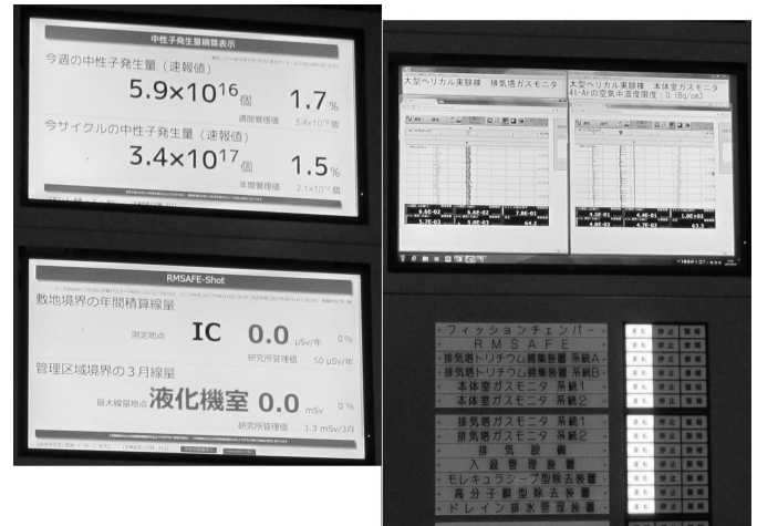
Figure 5: Three radiation monitoring displays and the interlock status indicator (right bottom): Top three screens usually show weekly and yearly neutron yield, plasma derived yearly and three-month cumulative doses (Sv), and gas radioactivity concentration ( \text{Bq}/\text{cm}^3 ) at the exhaust tower and the torus hall, respectively.
