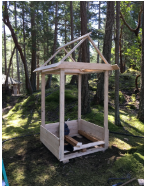
Figure 4.4. Roof and wall frames complete. Photo by David Chang 2018.
