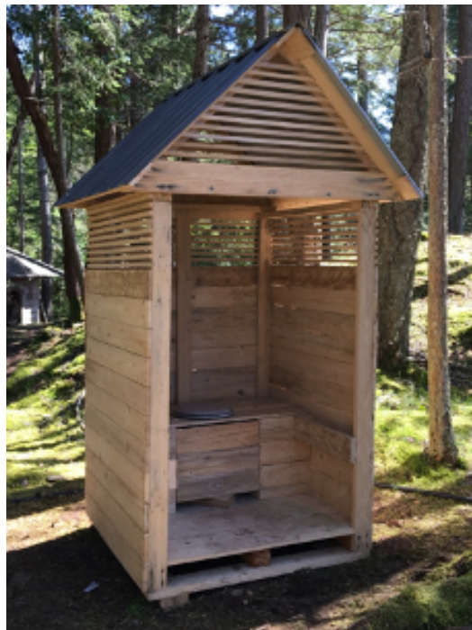
Figure 4.6. Completed outhouse. Photo by David Chang 2018.
